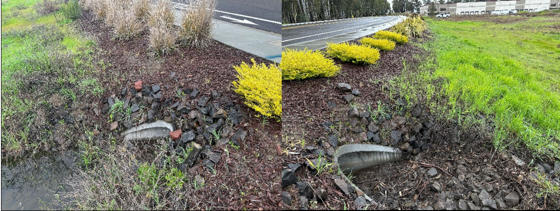
Photo 19: Storm drain outlet near southeastern corner.
