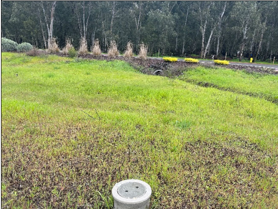
Photo 21: Electrical access hole inset about 30 feet from southeastern corner of site.
