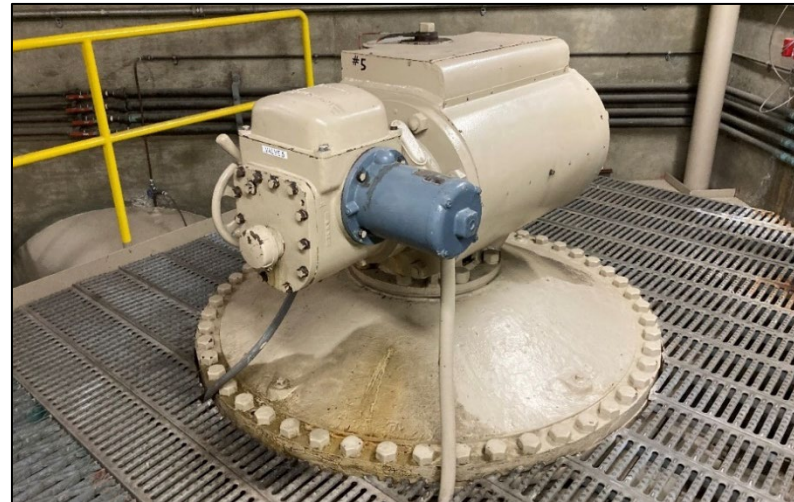
Valve Inside Junction Structure.
