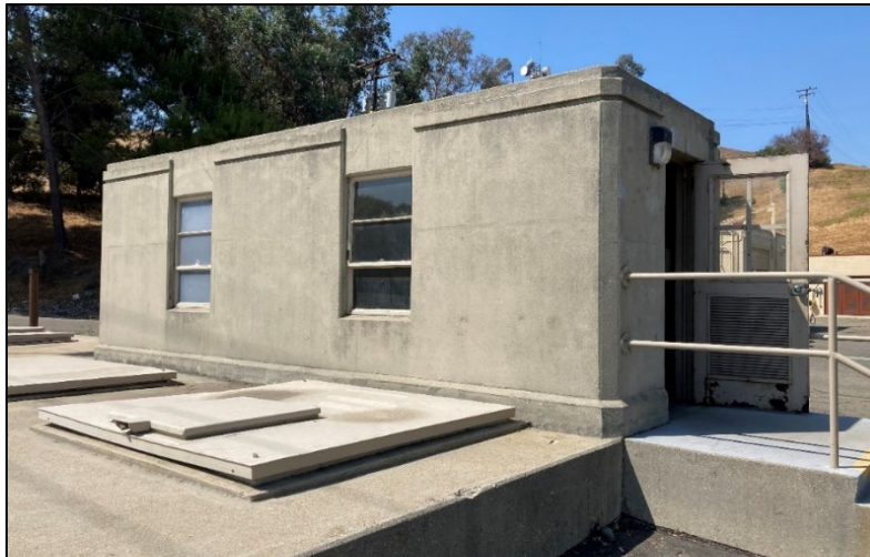
Eastern Elevation of Junction Structure, Facing South.
