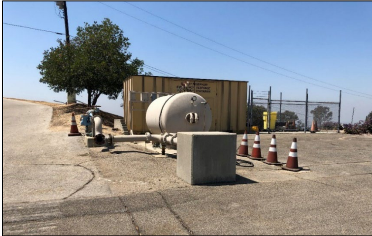
Surge Tank, Facing South
