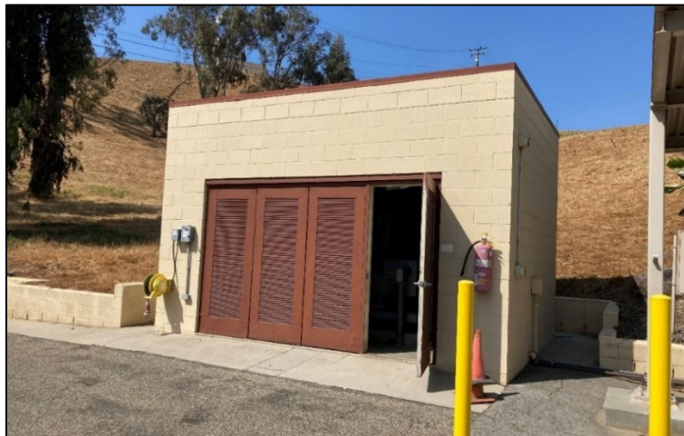
Standby Generator Building, Facing Southwest
