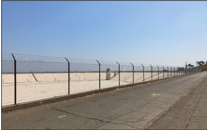
Reservoir, Facing Northeast.
