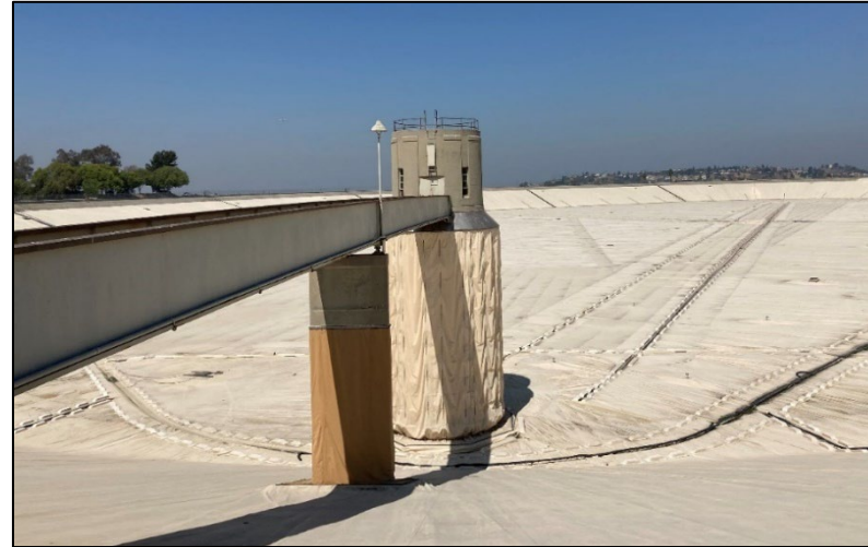
I/O Tower and Access Bridge, Facing West.
