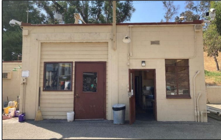
Northern Elevation of Administration Building and Water Quality Laboratory, Facing South
