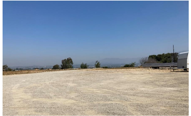
Photograph 8. Construction Staging Area
