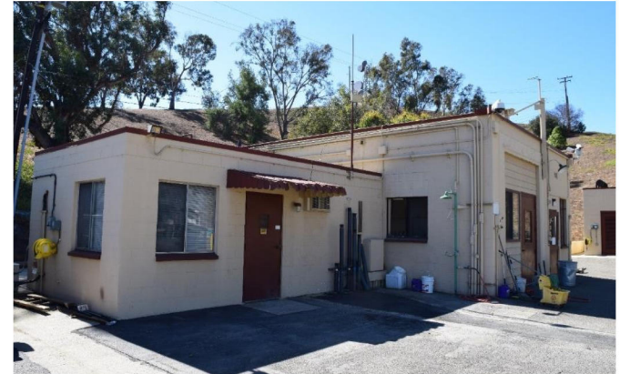
Photograph 4. Administration Building and Water Quality Laboratory
