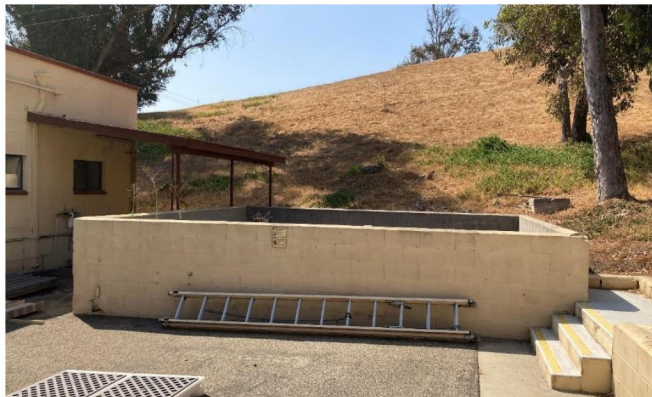
Photograph 5. Former Caustic Soda Structure
