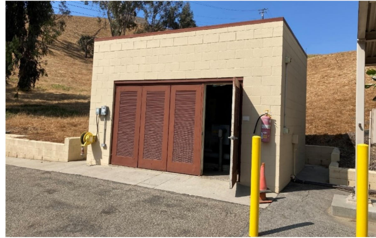
Photograph 2. Backup Generator Enclosure
