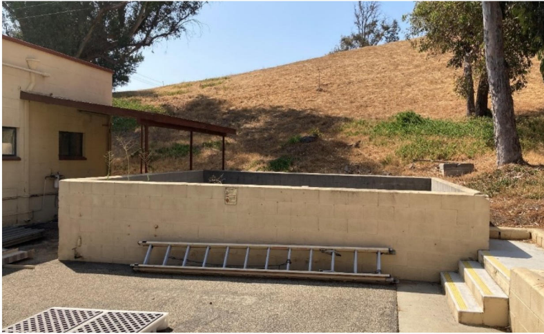
Photograph 1. Former Caustic Soda Structure
