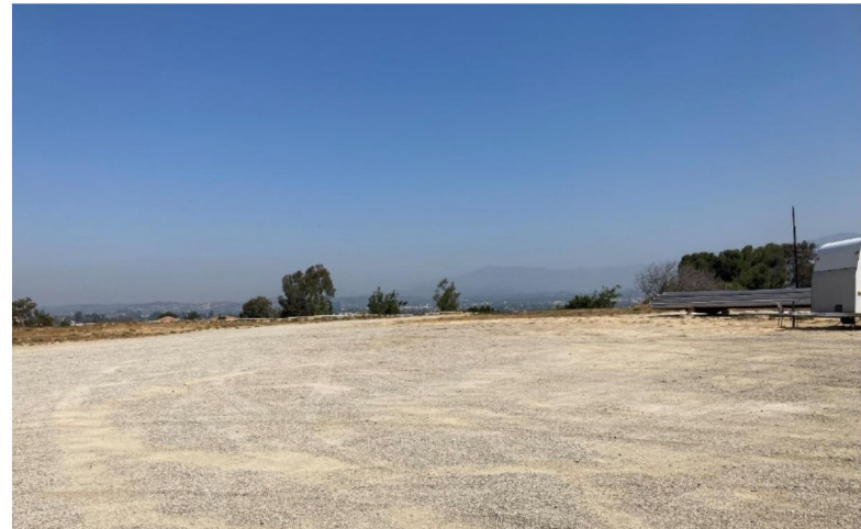
Photograph 4. Construction Staging Area
