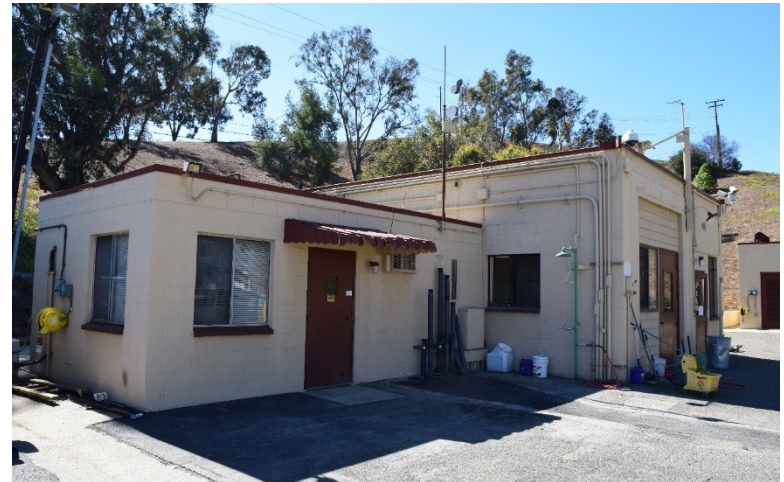
Photograph 4. Administration Building and Water Quality Laboratory
