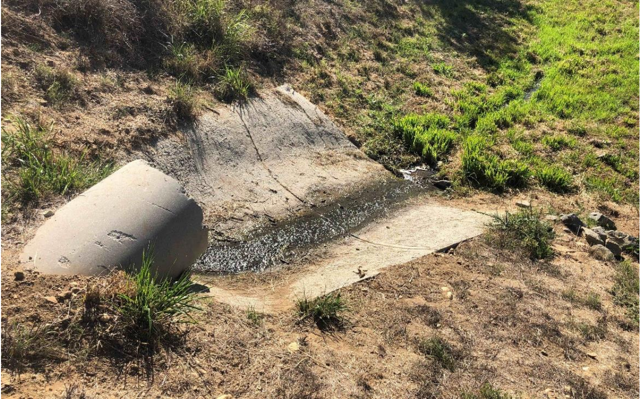
Photograph 7. Culvert outlet conveying flow from Basin 1 to Basin 2, facing southeast.
