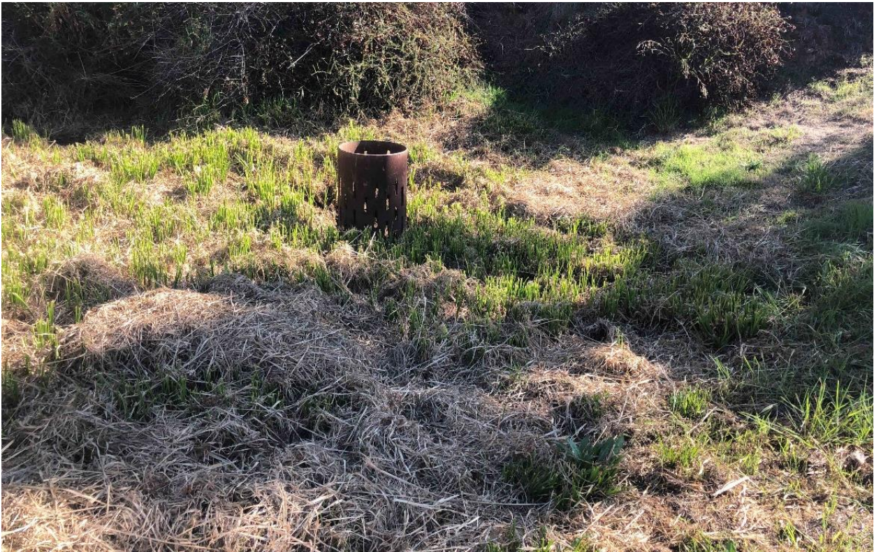
Photograph 4. Inlet drain receiving flow from Basin 1, facing east.
