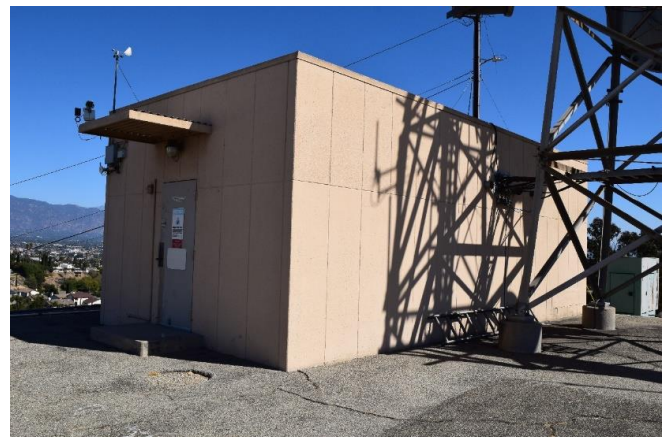
Photograph 12. Building at Communications Site
