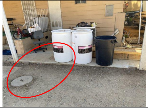
View of septic system at rear side of 26399 address with two empty 55-gallon drums
