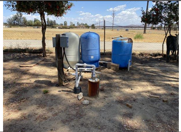
View of the waterwell
