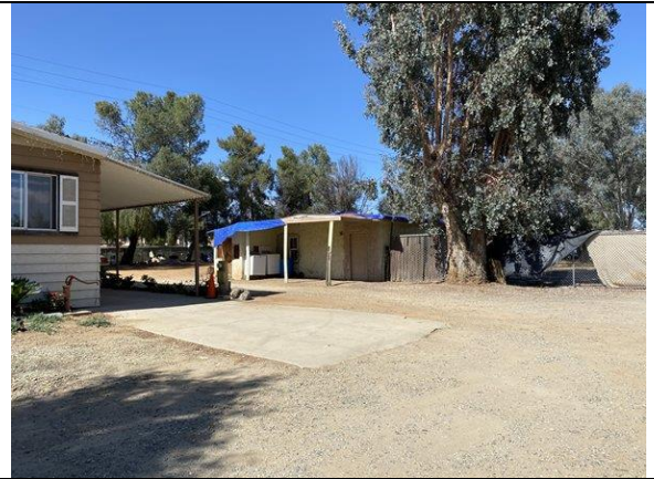
View of outbuilding- used for storage by rear side of 26429 building
