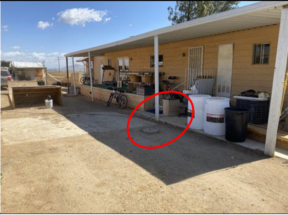
View of rear side of 26399 building
