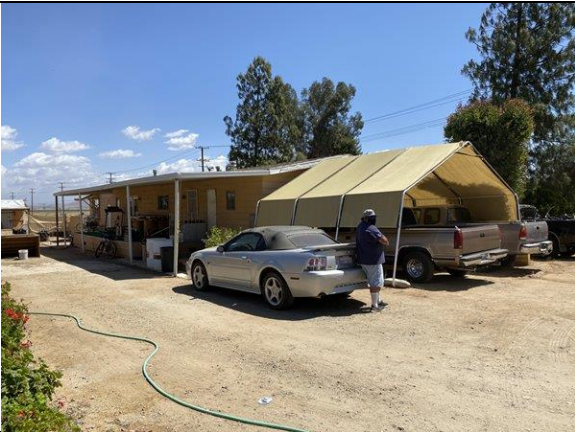
View of the 26399 mobile home building to the north side of the Property along Murrieta Raod
