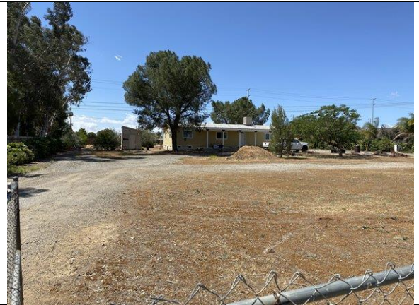
View of the Property – 25981 Elm Street
