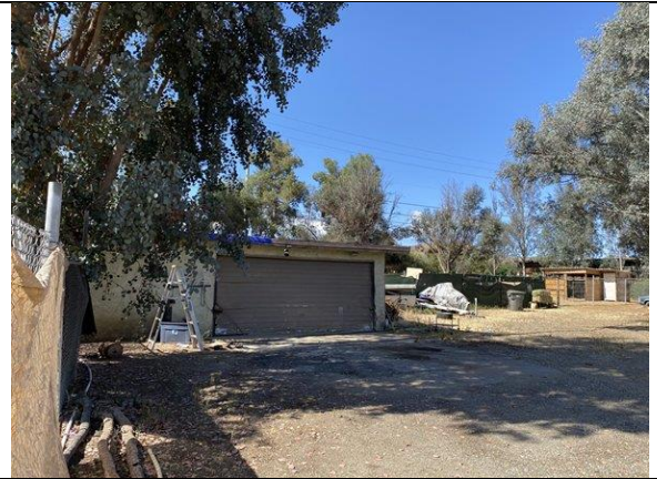
View of garage - tools storage
