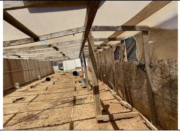
View of former grow area located rear side of Property
