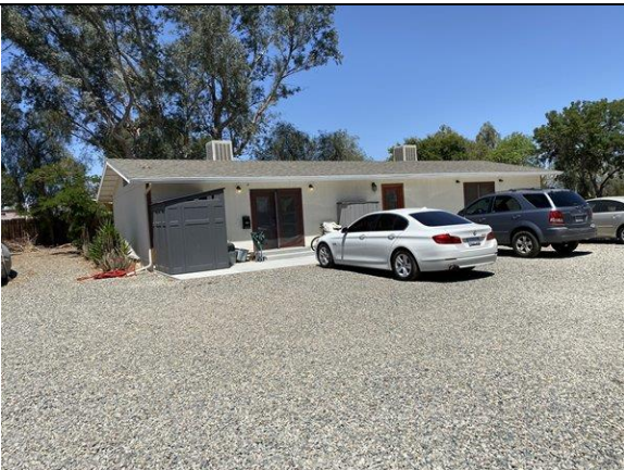
View of mobile homes at 25931 Elm Street
