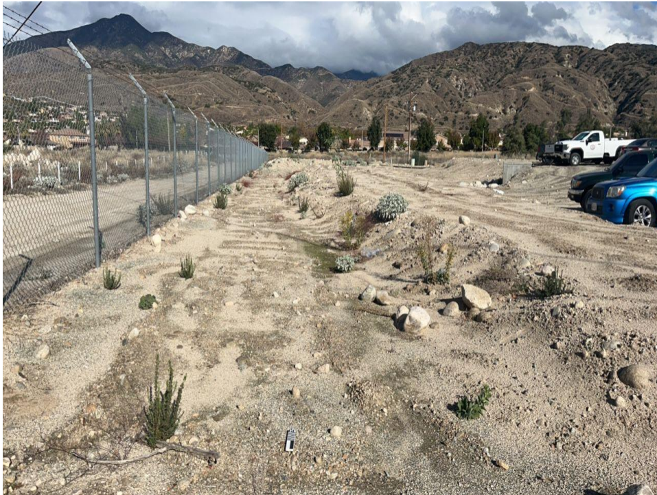
Figure 4. General View along Northwest Chain-Link Fence, View NW
