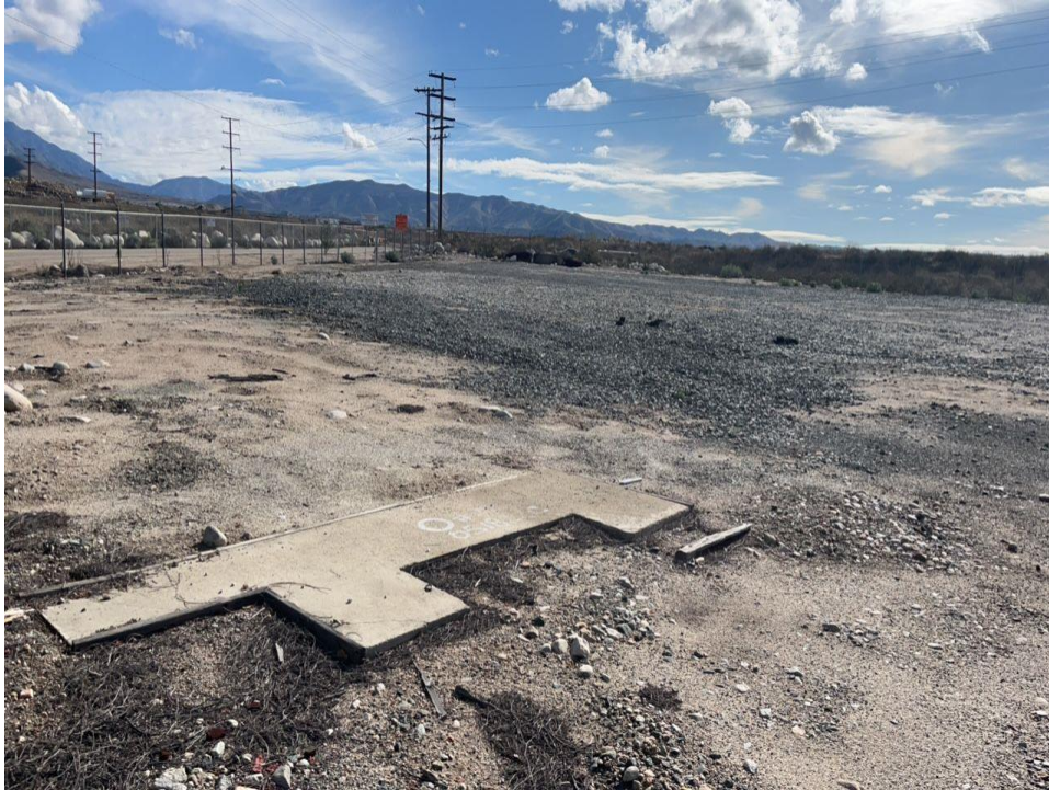
Figure 8. Overview F-Shape Poured Cement Foundation, View SW
