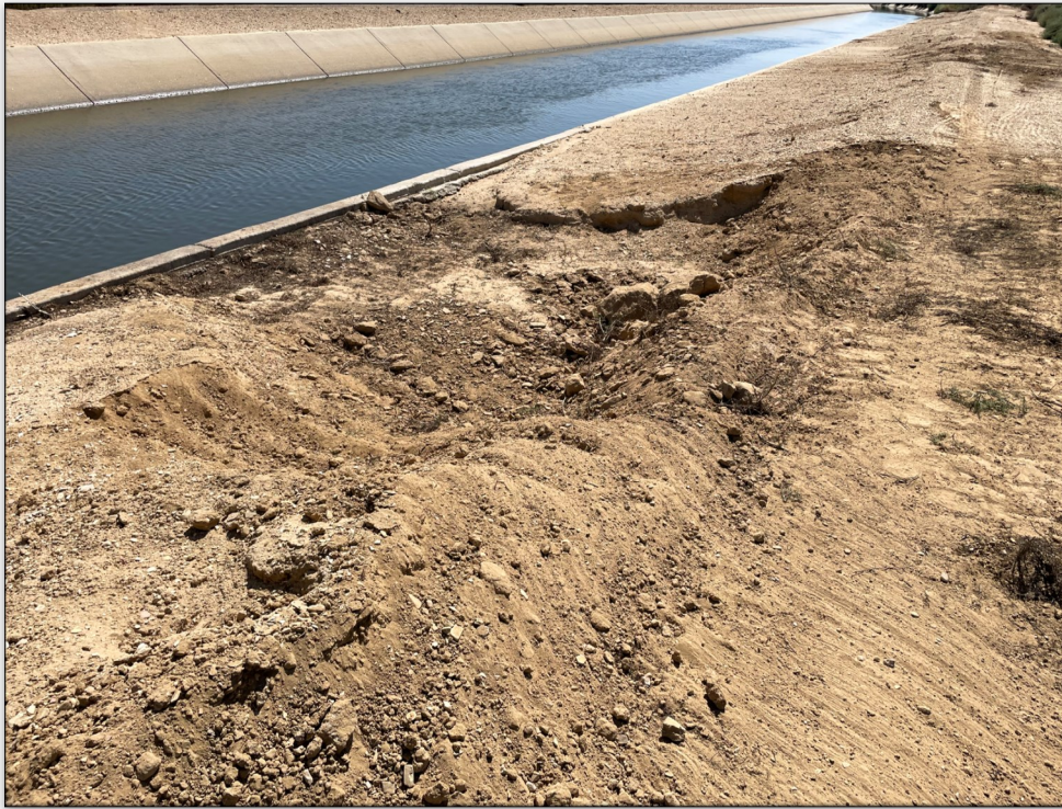
Photograph 17 Overview of 500 Construction Area 1.
