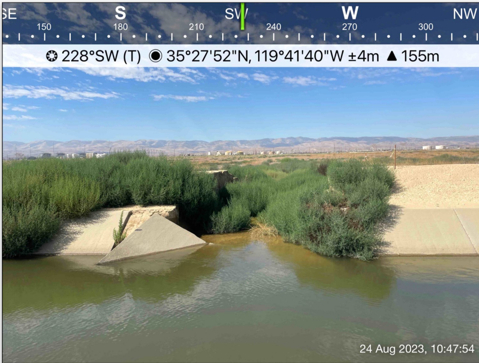
Photograph 18 Overview of 500 Construction Area 2.
