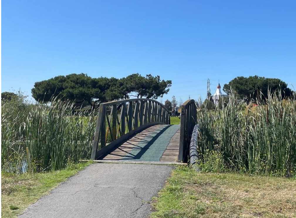
Photo 3. View of Existing City Bridge #27 looking south.
