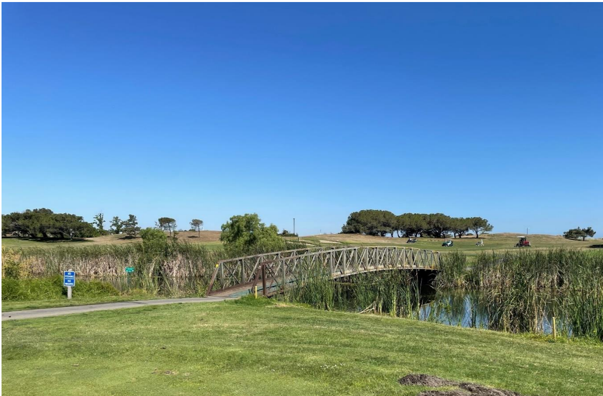
Photo 4. View of Existing City Bridge #27 looking northwest.
