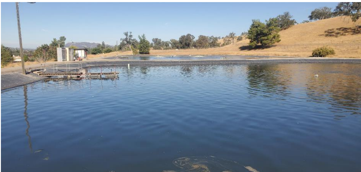
Photograph 2. Photograph of the existing wastewater treatment plant, facing northwest. October 6, 2022.
