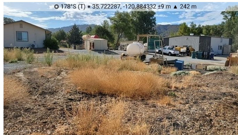
Photograph 2. Existing HRCSD Wastewater Treatment Plant Support Structures, Facing South.
