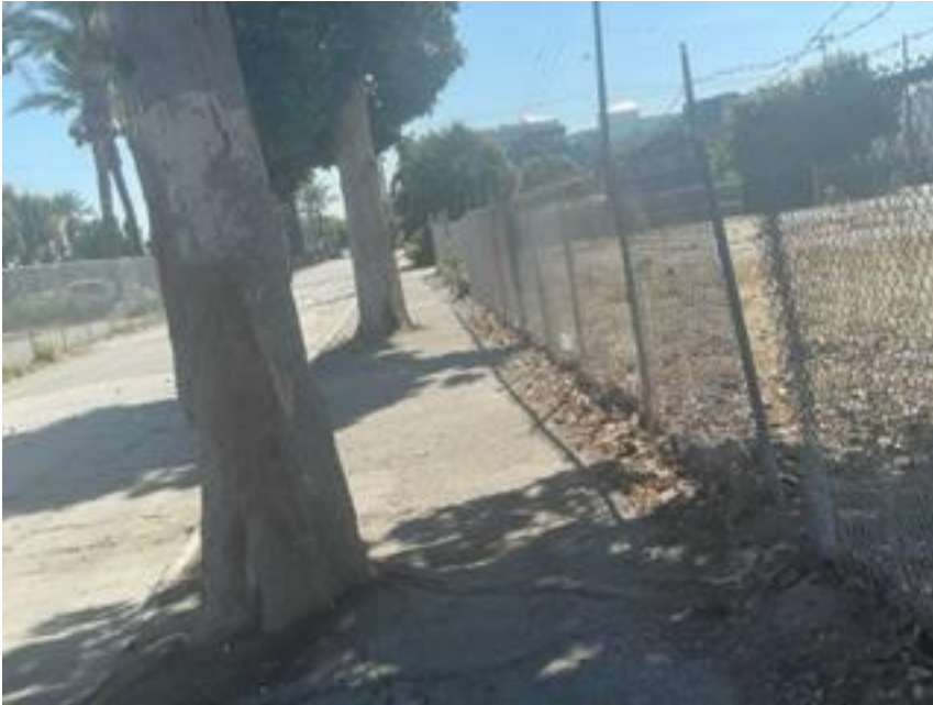
Trunks of tree numbers 2 and 3 with their root crowns paved up to with concrete sidewalks and curbs.
