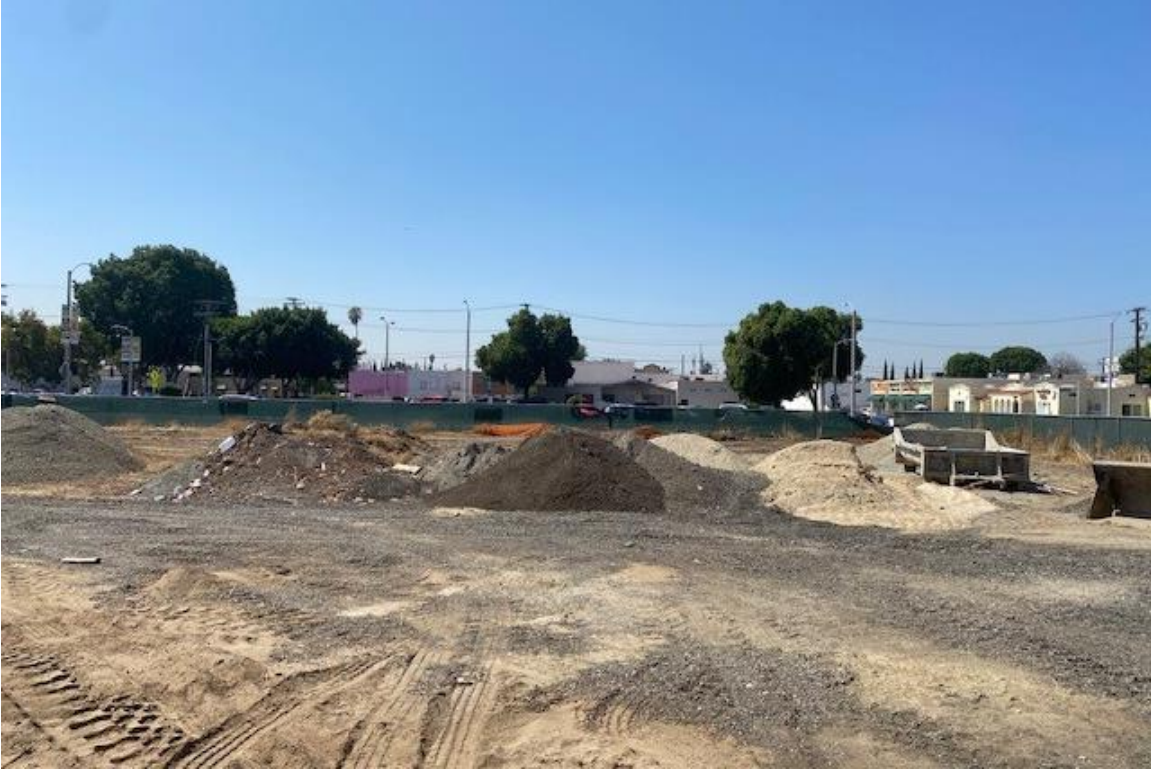
Figure 5 Overview of project area, including active construction, facing south
