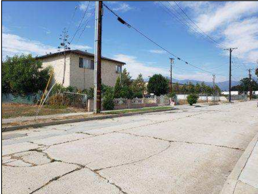
12 : Looking northwest of the adjoining residential home bisecting the northwest and southwest vacant lot.
