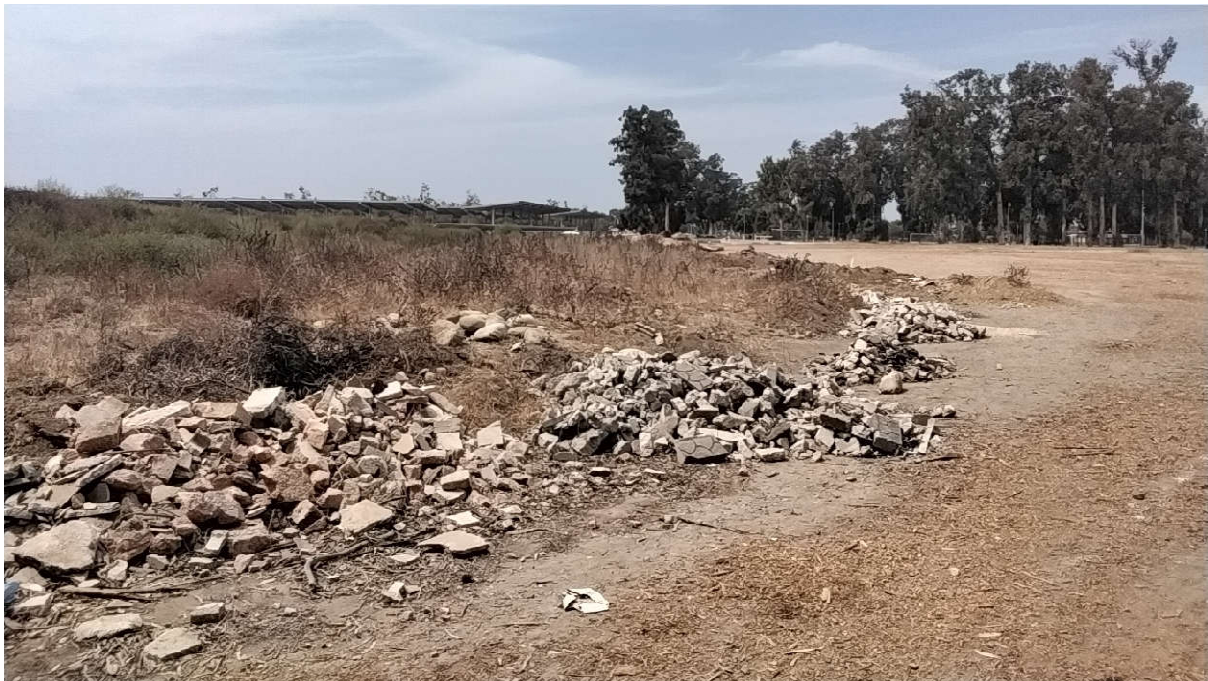
Photograph 2. View of five piles of concrete debris in the southeastern corner of the subject property, facing west.
