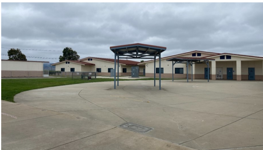
Overview of the buildings surrounding the Bonita Elementary School quad, view northwest.
