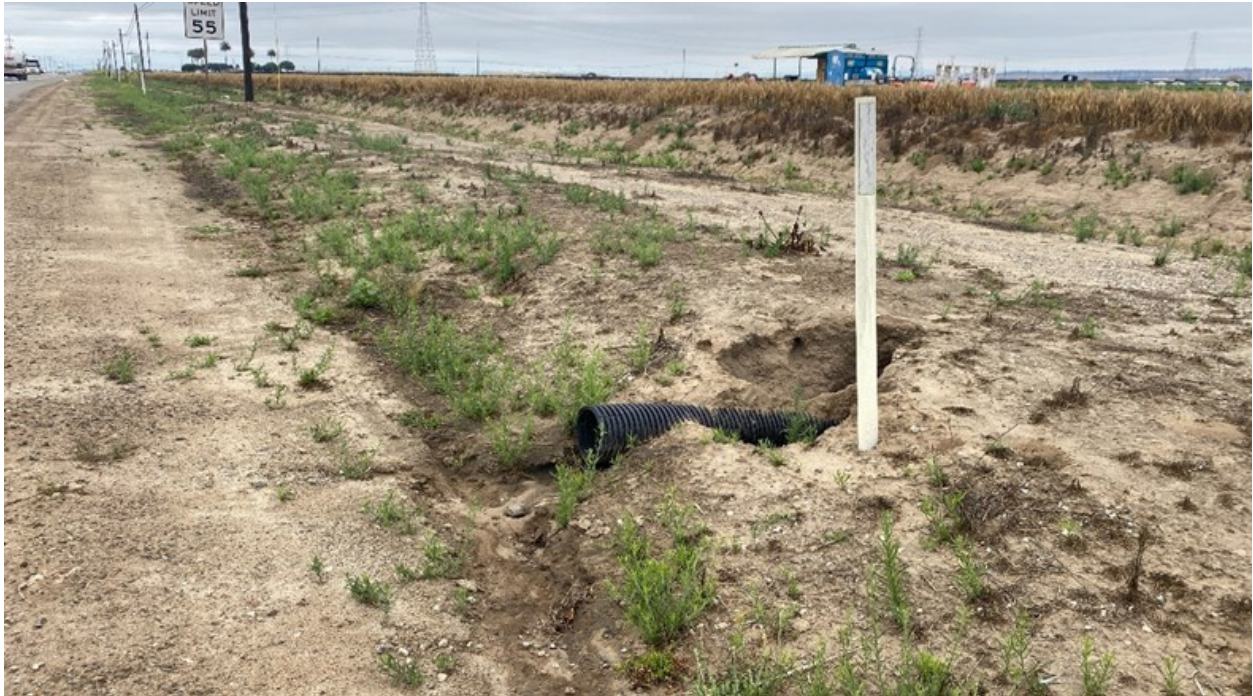
Photograph 1. South side of State Route (SR) 166, view east.
