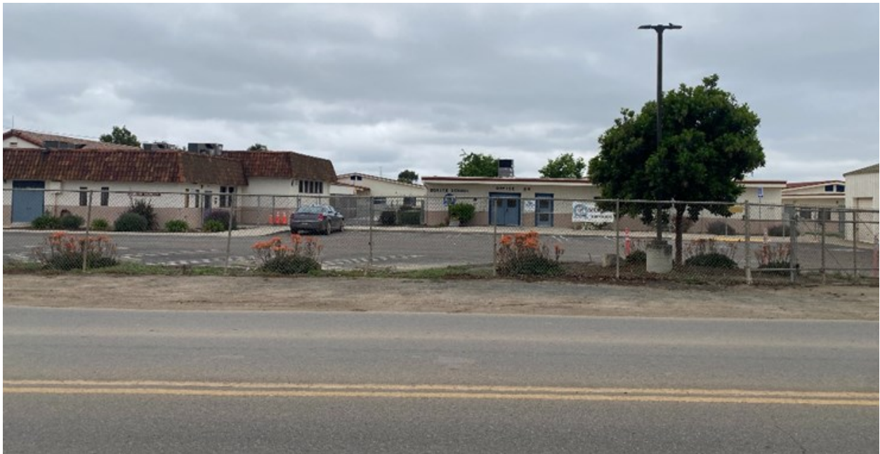
Photograph 6. Overview of Bonita Elementary School campus, view north.
