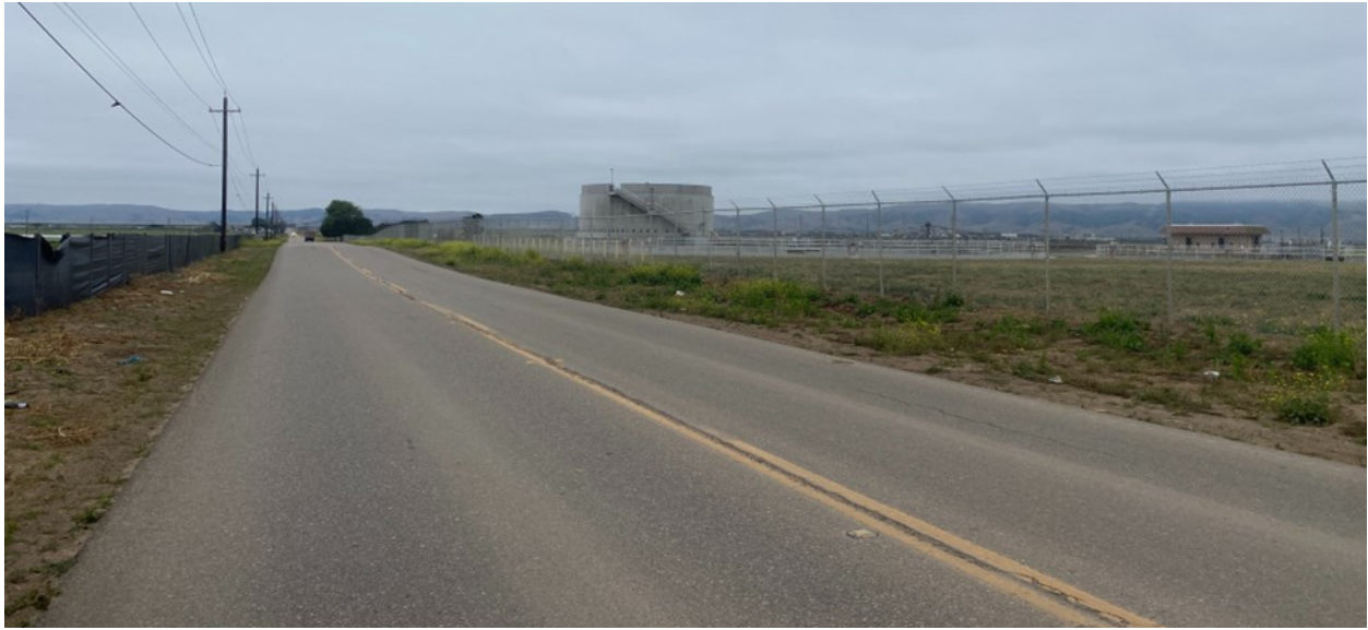
Photograph 3. Black Road, view north.
