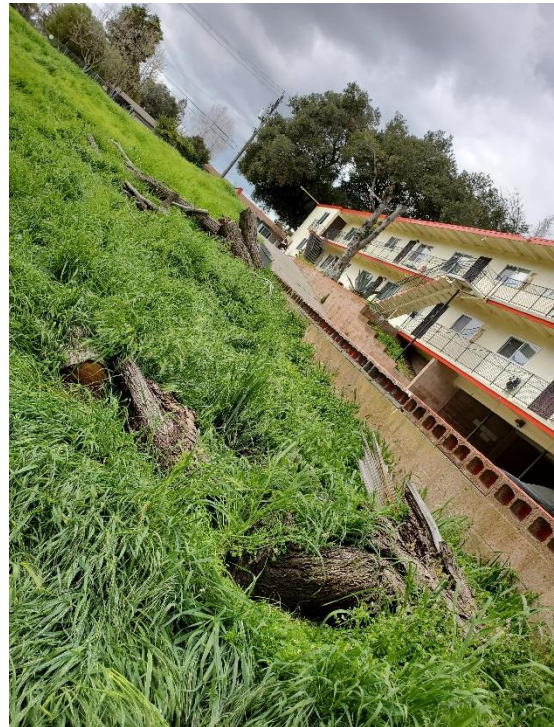
Figure 2. Portions of the trunk of tree #3 (background/top) were left in place, but not enough to directly measure the trunks. Both trunks of tree #4 (foreground) were on the ground right where they were felled, and diameter measurement where the trunk would be 54" above grade was possible.
