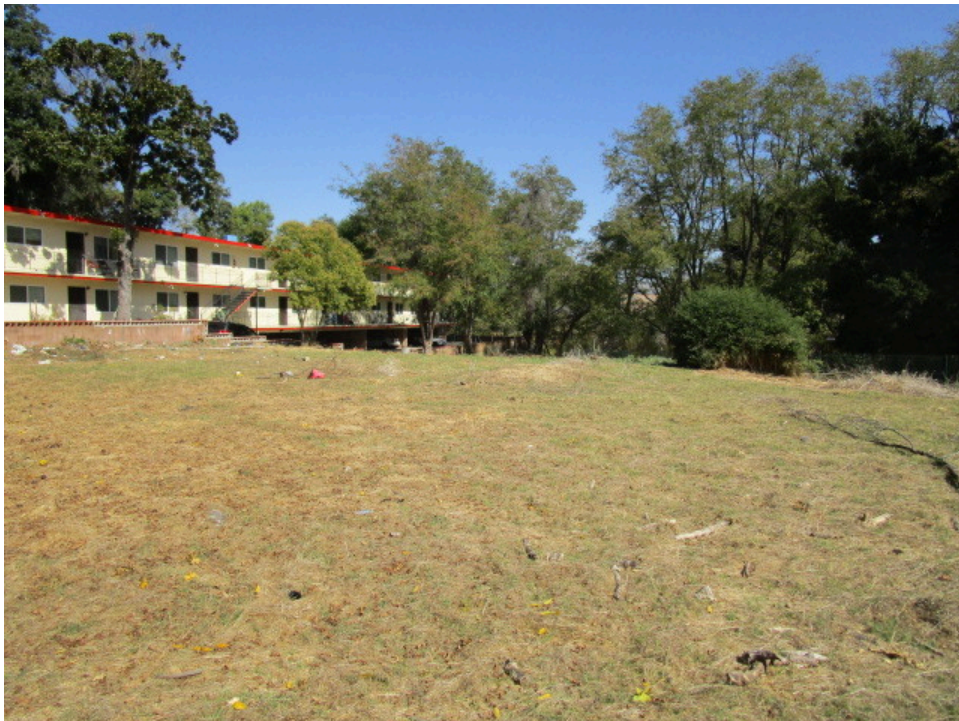
24. The subject property from its southwestern property line (3 of 5)
