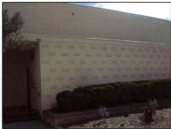
Detail of Entry on West Elevation
