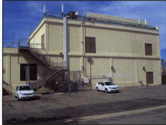
East (Rear) Elevation, Facing West/Northwest
