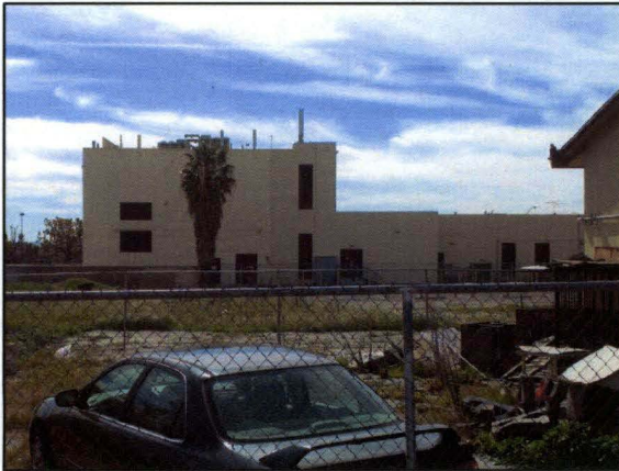
North Elevation, Facing South
