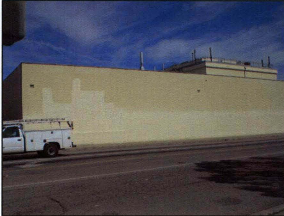
South Elevation, Facing Northeast
