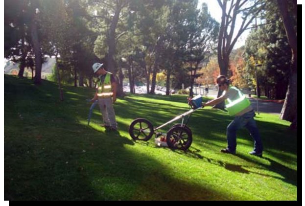
Ground Penetrating Radar and 50/60HZ
