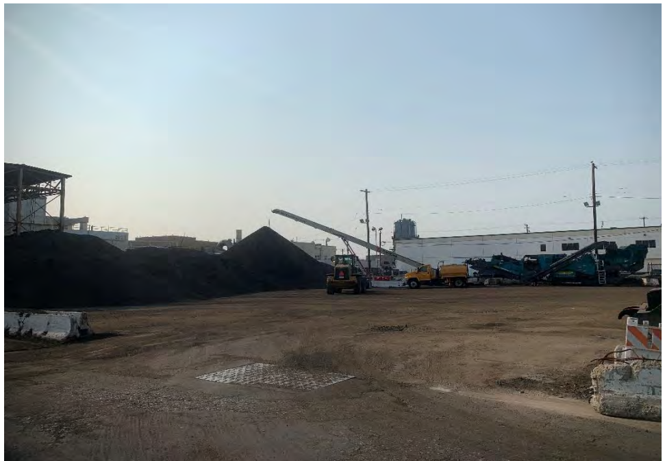
Photograph 4: On alleyway, looking southeast at the site.
