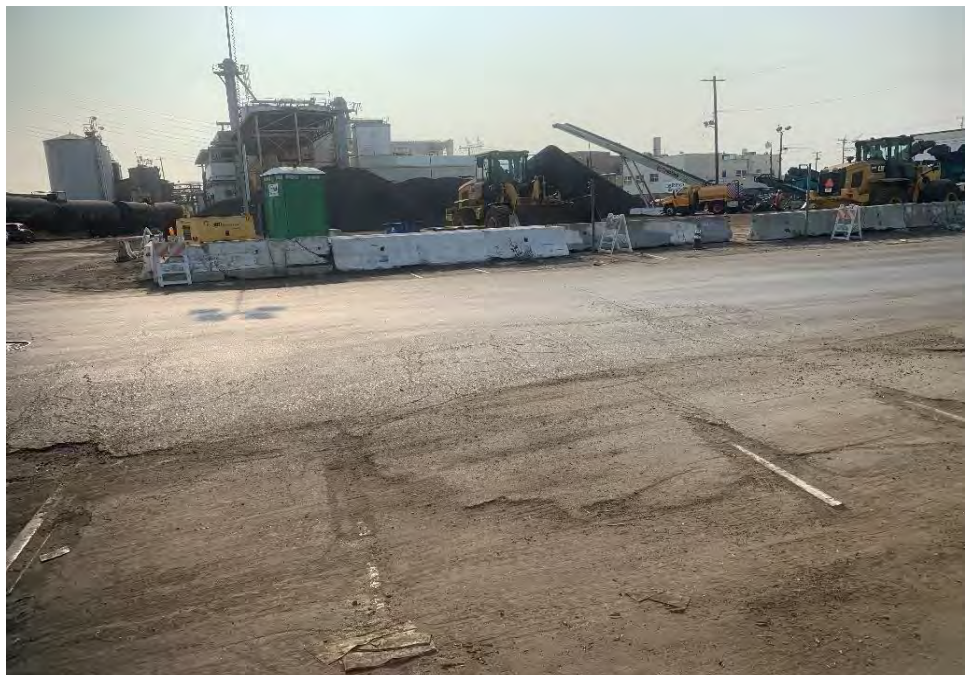
Photograph 6: View of buried railroad tracks, followed by Harriet Street and the site looking east.
