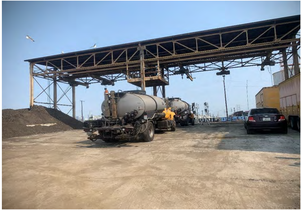
Photograph 7: On the southern end of the concrete platform looking north at the site with view of metal canopy and supports.
