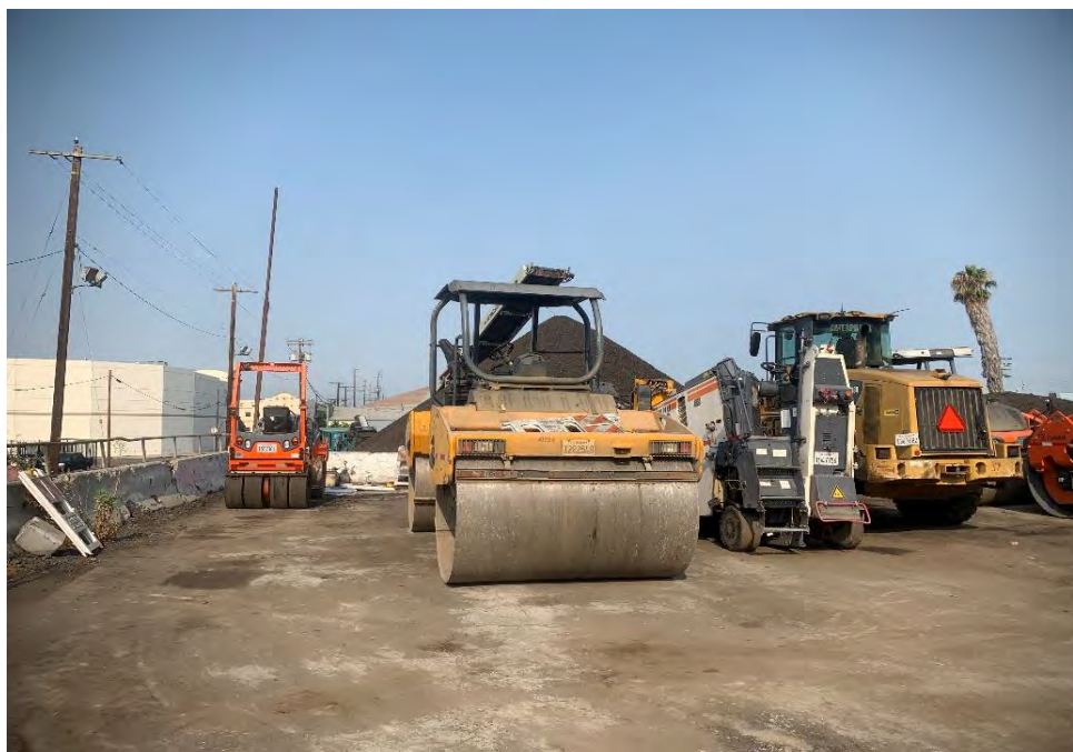
Photograph 2: Southern portion of concrete pad looking west at the site.
