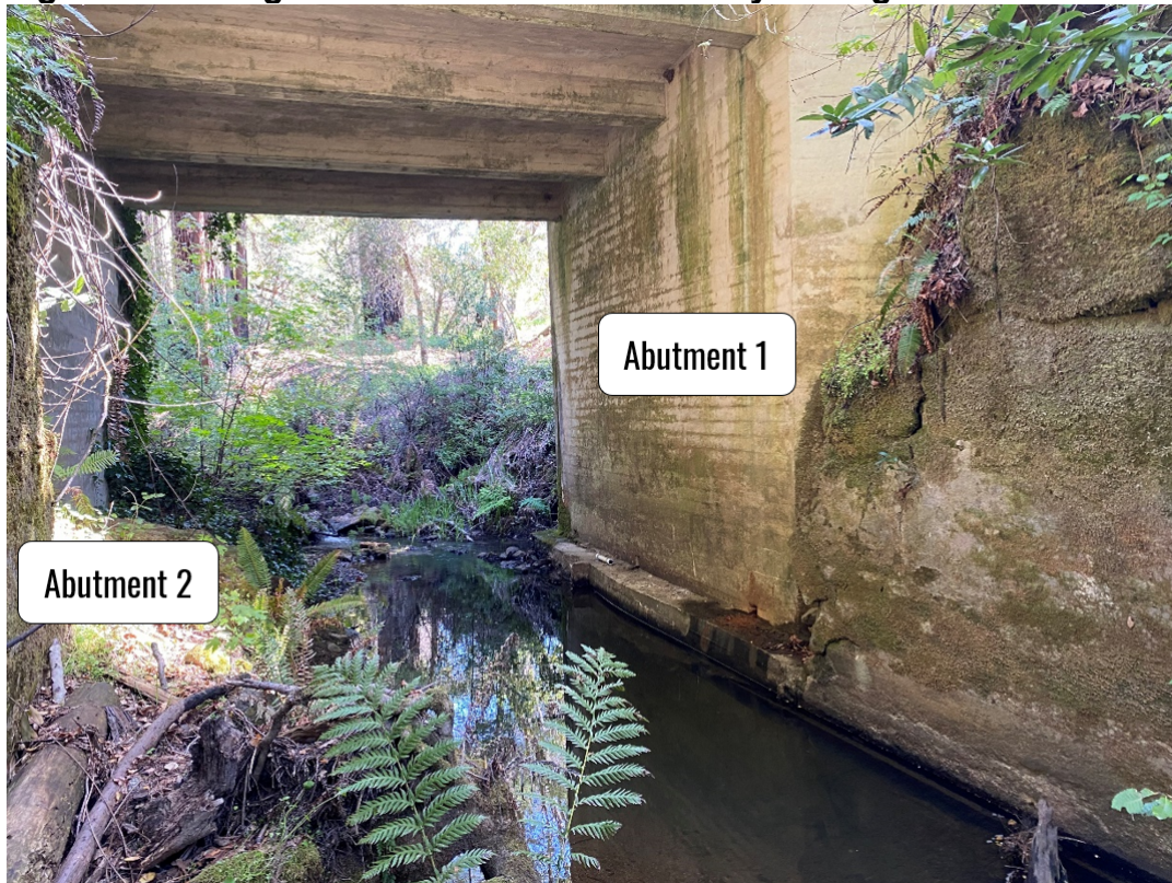
Figure 1-6 Bridge Abutments Under Roadway Facing South
