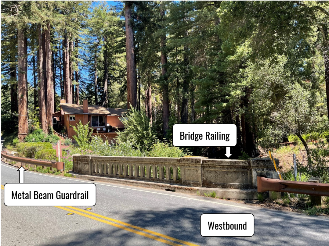
Figure 1-4 Boulder Creek Bridge on State Route 236 Facing Northwest
