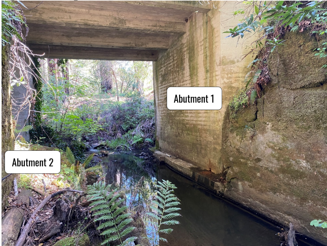
Figure 1-6 Bridge Abutments Under Roadway Facing South
