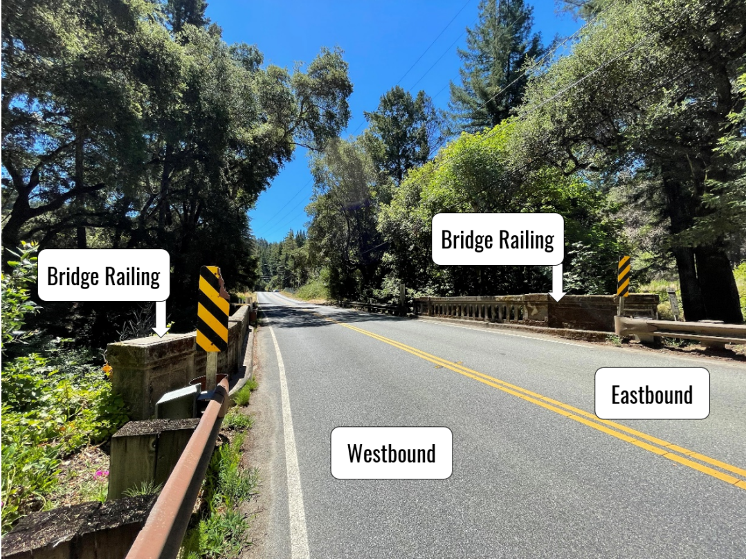
Figure 1-3 Boulder Creek Bridge on State Route 236 Facing Southeast
