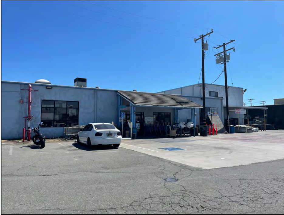
View southwest of the north elevation.
