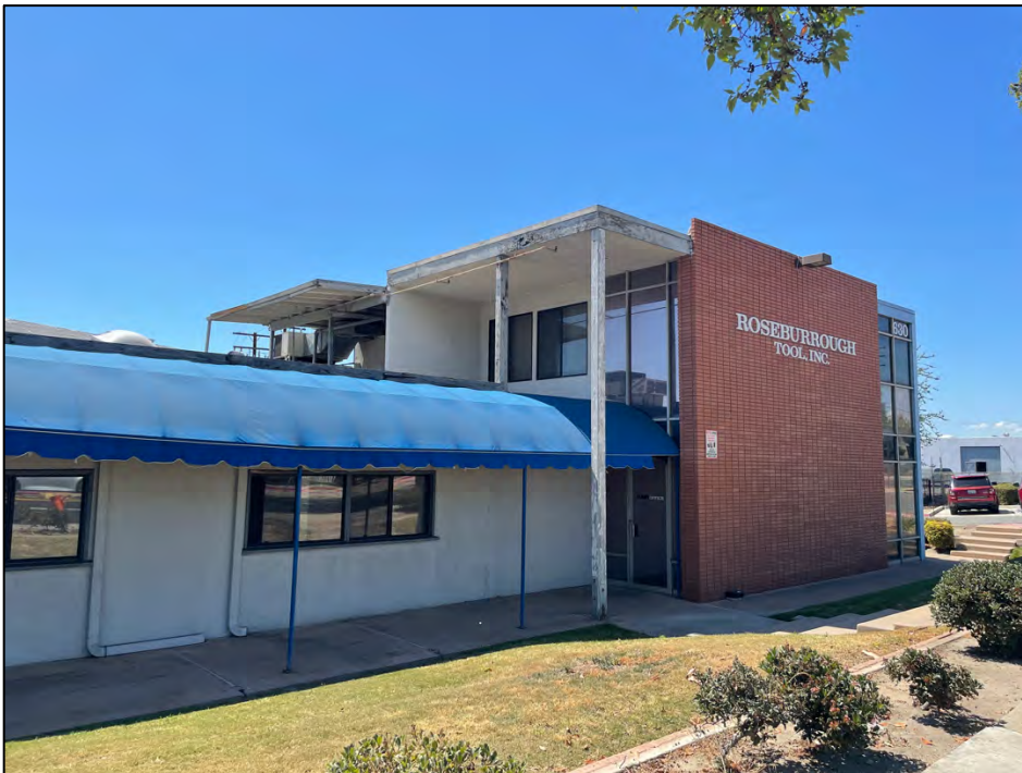
View northwest of the main elevation from Batavia Street.
