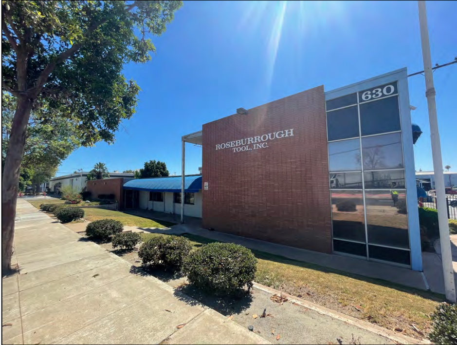
View southwest of the main elevation from Batavia Street.
