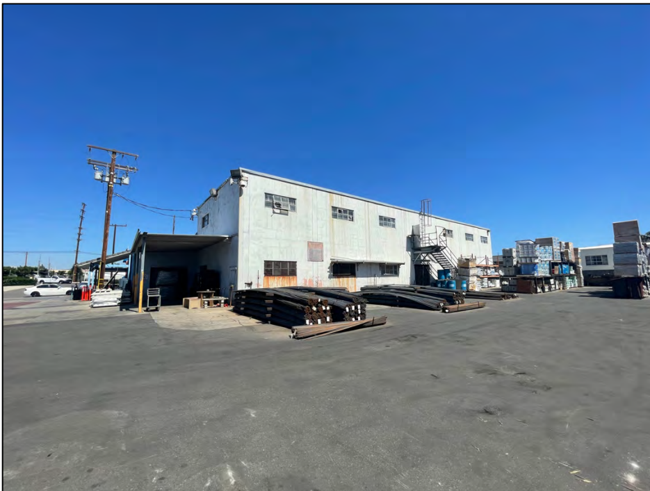
View east of the west elevation and partial north elevation.
