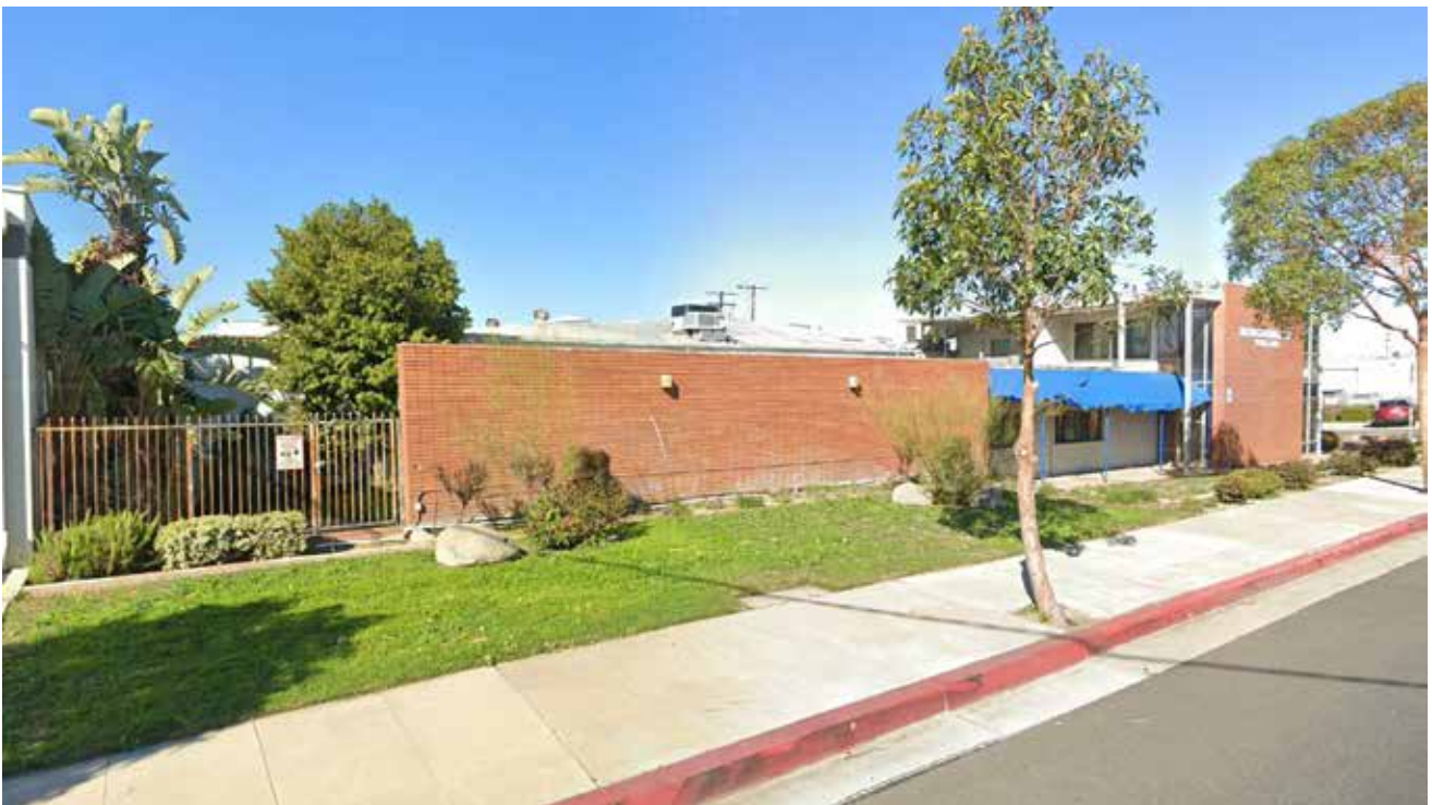
Existing structure viewed from Batavia St.
