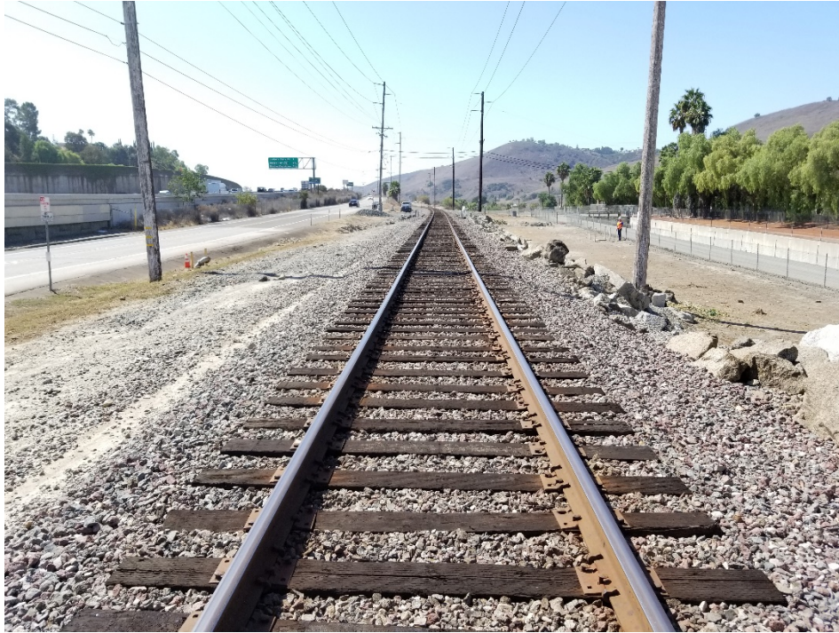
Figure 1. Overview of Segment 1 of P-19-186804 / P-30-176663 facing south.
