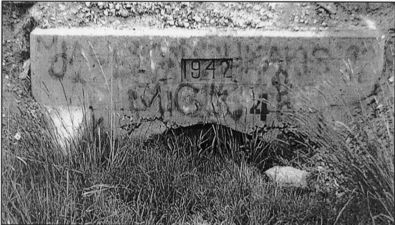
Old concrete culvert across the railroad bed
