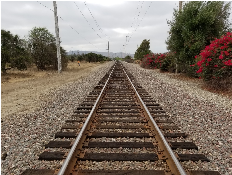
Figure 2. Overview of Segment 2 of P-19-186804 / P-30-176663 facing south.
