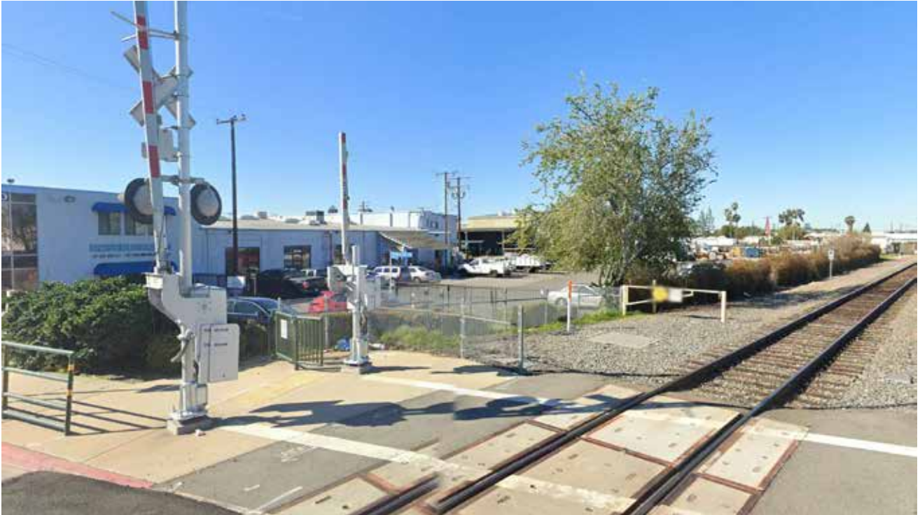
View from the northeast corner of project site at the railroad crossing on Batavia St.
