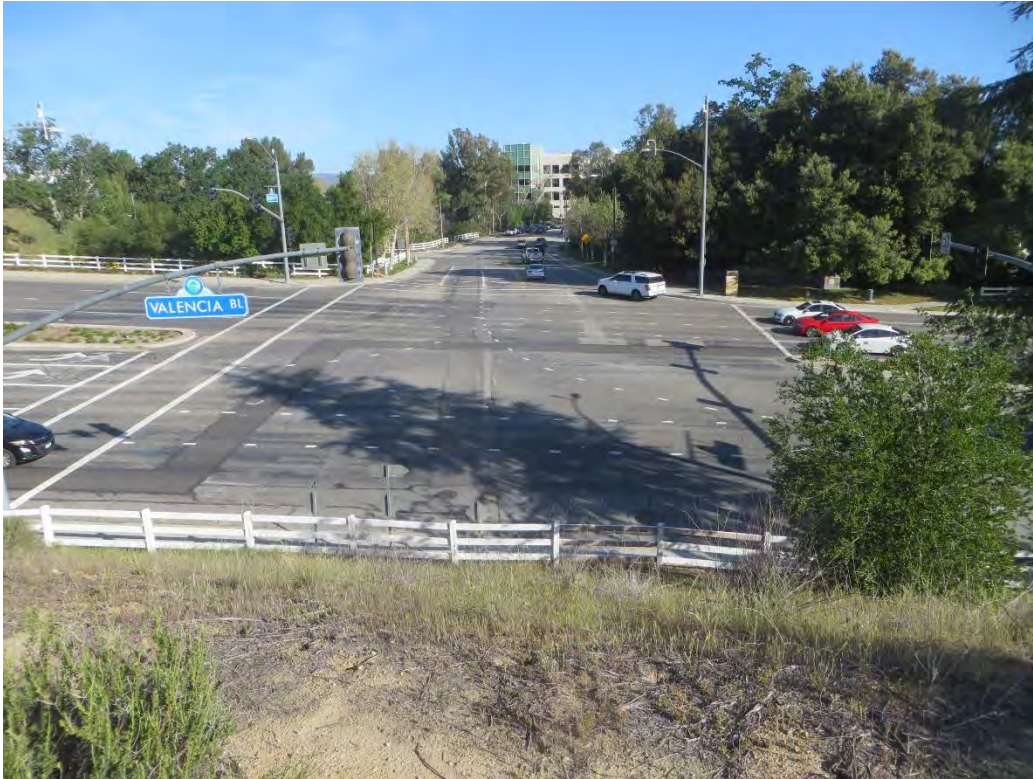
Photograph 3: North-facing view of the intersection of Valencia Boulevard and Tourney Road.
