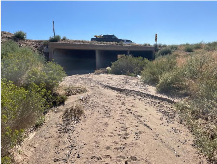
**Photo 6.** View of box culvert along the southeastern portion of the project site, which conveys flows underneath Mojave Drive along NWW- 03. Facing northeast.
