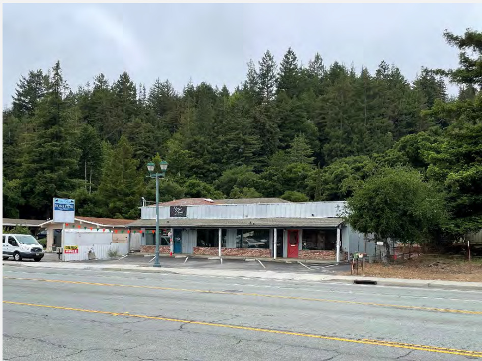
Exhibit 1. Main (east) elevation of the Business Complex (A), facing southeast (Image_1509).
