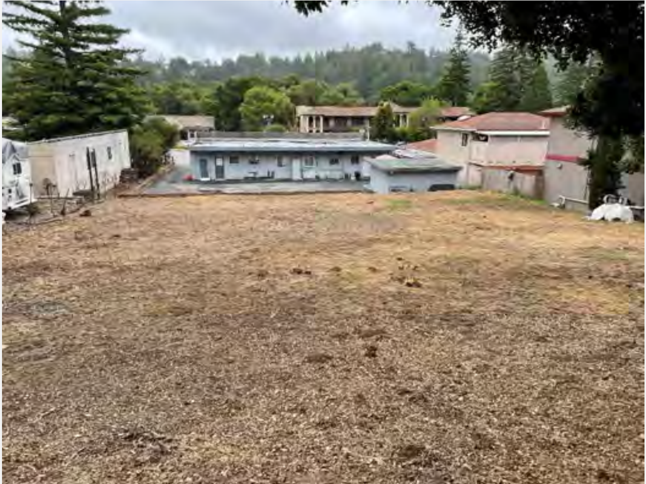
Exhibit 2. View of the grass field, Outbuilding (B), and rear (west) elevation of the Business Complex (A) from the west boundary of the property. View looking east (Image_1498).
