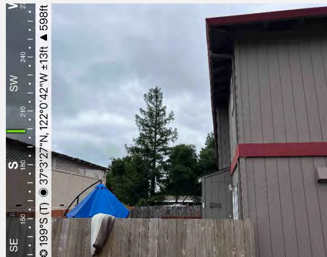
Photo 4. Photo of structures at the western edge of the Project site, with marginal roosting bat habitat.
