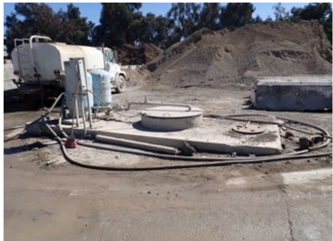
9. View of water well located near east-central portion of property.
