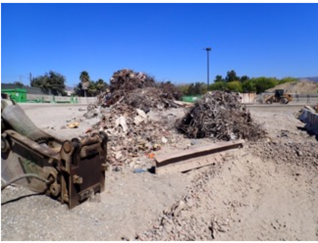
7. View of waste metal debris piles near center of property.
