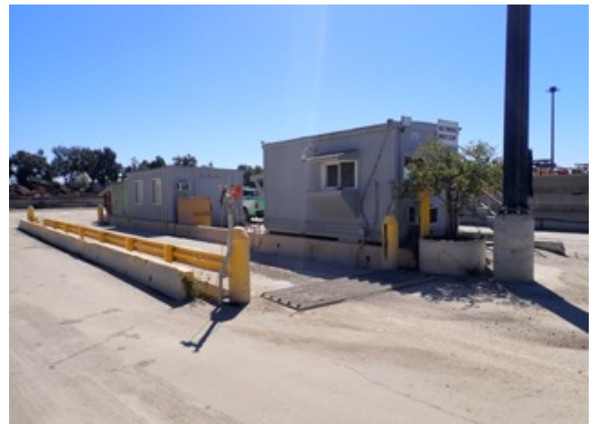
10. View of the two small office & breakroom container structures, looking southeasterly.
