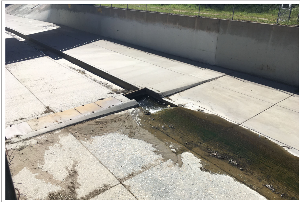
Photo Location 3. February 10, 2022. View of diversion structure in the mainstem Arroyo Seco channel.
