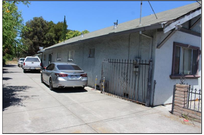
2. View of the subject property featuring one of the 1271 East Julian residential building with a concrete-paved driveway.
