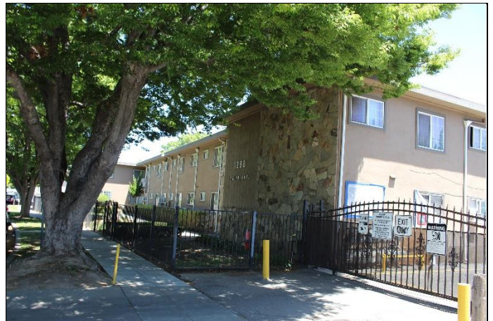
24. View of the adjacent residential apartment buildings located to the northwest.
