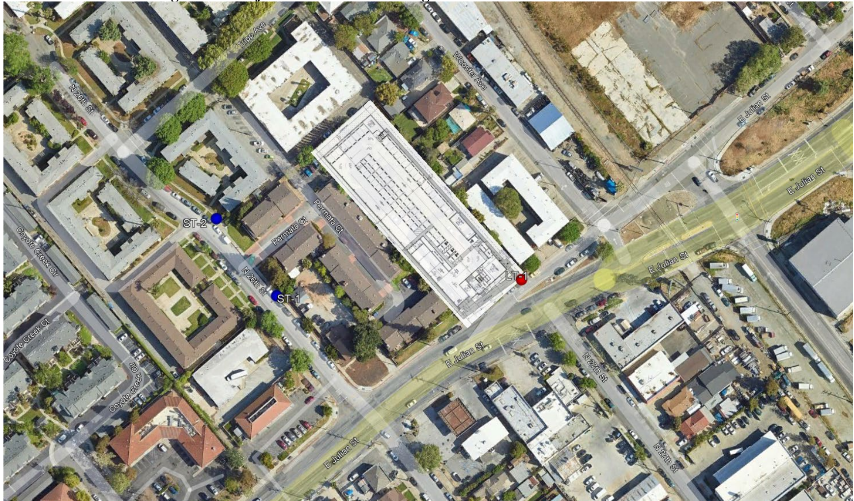
FIGURE 1 Aerial Image of the Project Site and Surrounding Area with the Noise Measurement Locations Identified
