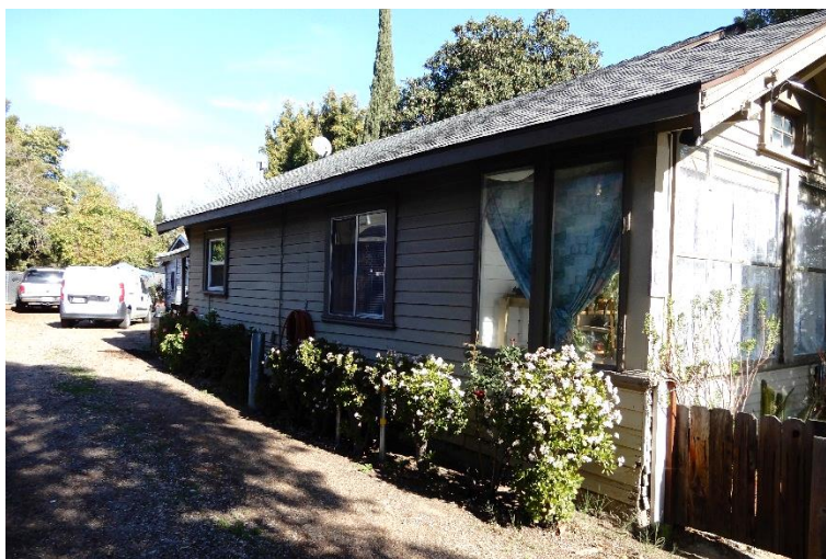
Figure 5. 1279 E. Julian Street, west façade, view northeast (ARG, March 2021)
