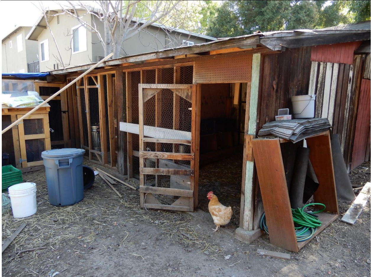
1279 E. Julian Street, one-story structure, north façade, view southeast (ARG, March 2021)
