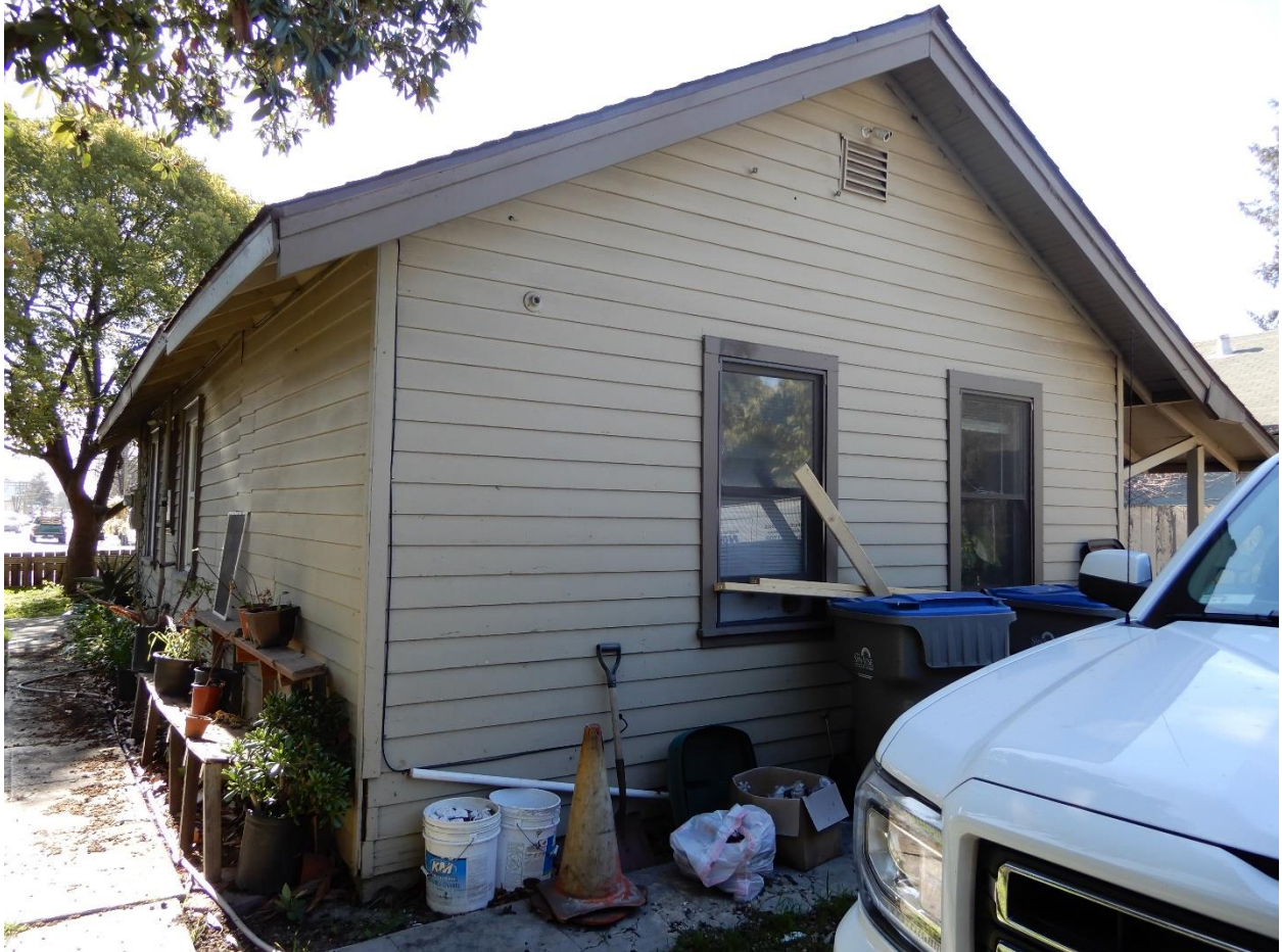
1279 E. Julian Street, rear (north) façade, view southwest (ARG, March 2021)
