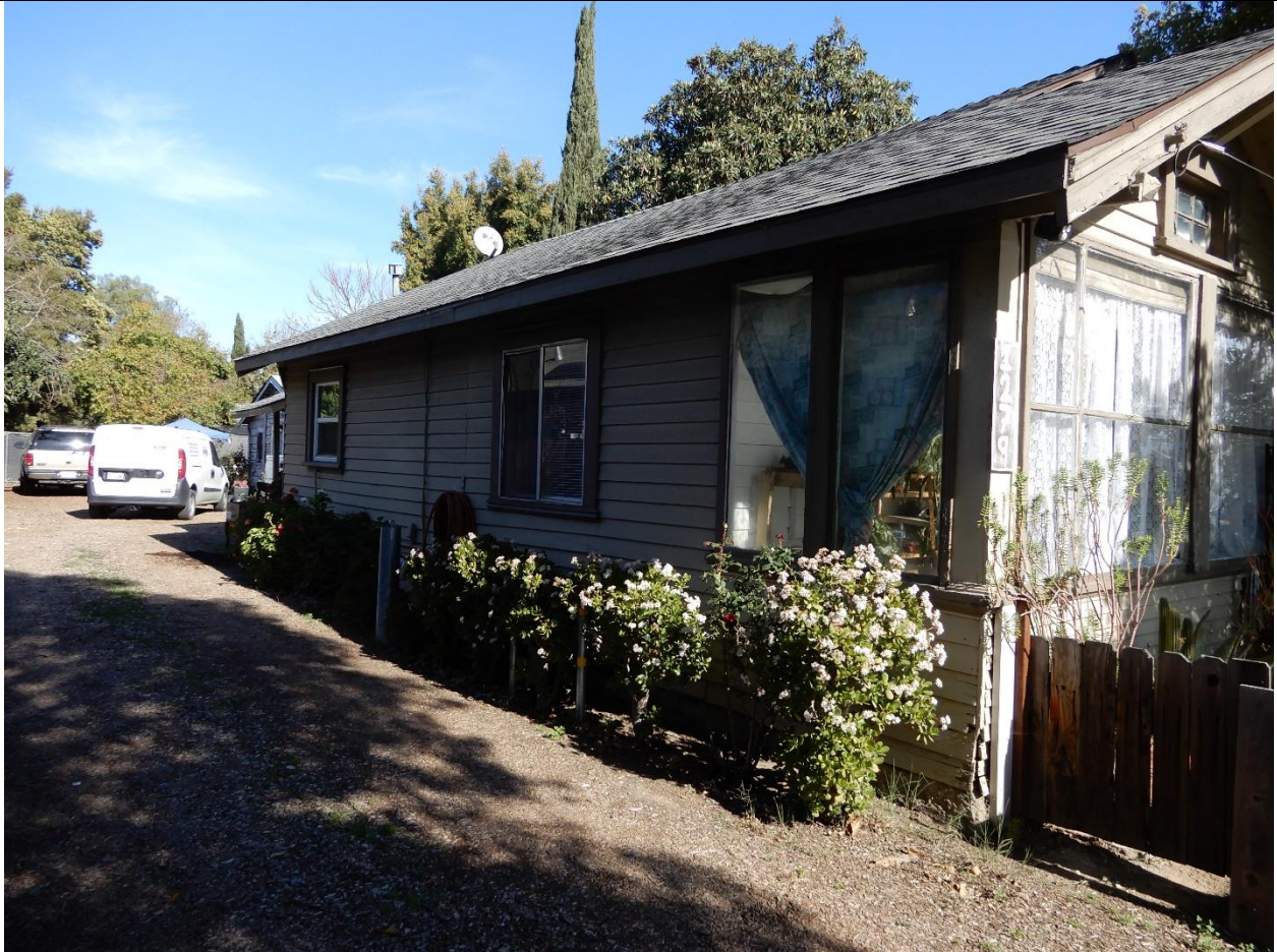
1279 E. Julian Street, west façade, view northeast (ARG, March 2021)
