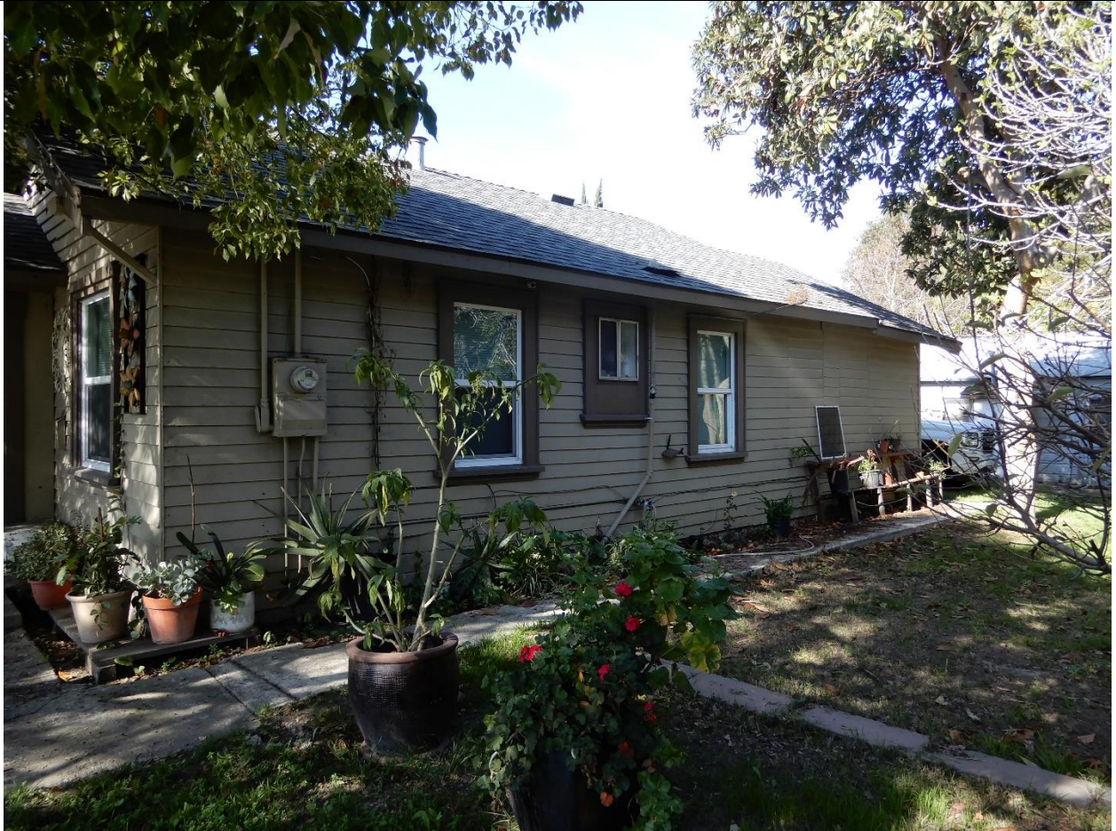
1279 E. Julian Street, east façade, view northwest (ARG, March 2021)
