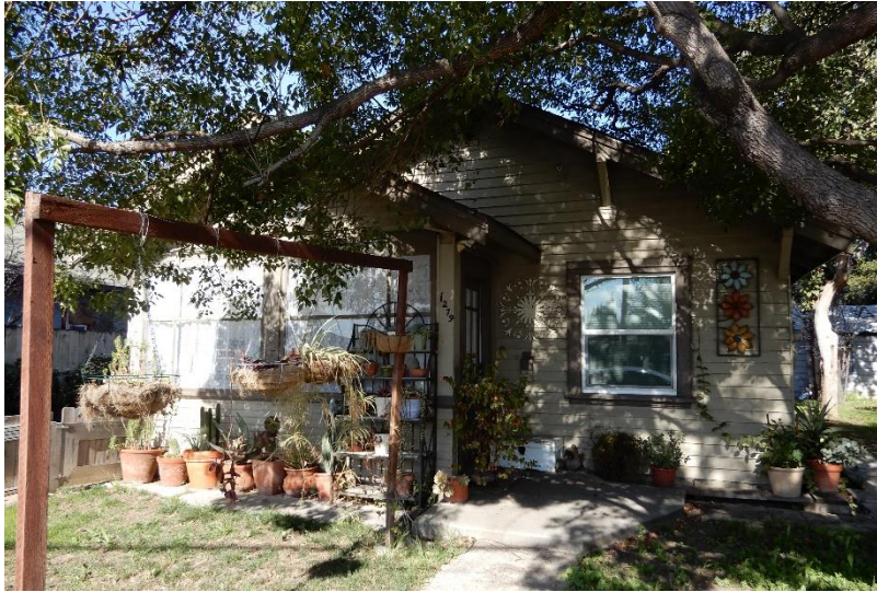
Figure 4. 1279 E. Julian Street, primary (south) façade, view northwest (ARG, March 2021)
