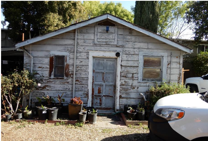
Figure 6. One-story residential building behind 1279 E. Julian Street, west façade, view east (ARG, March 2021)
