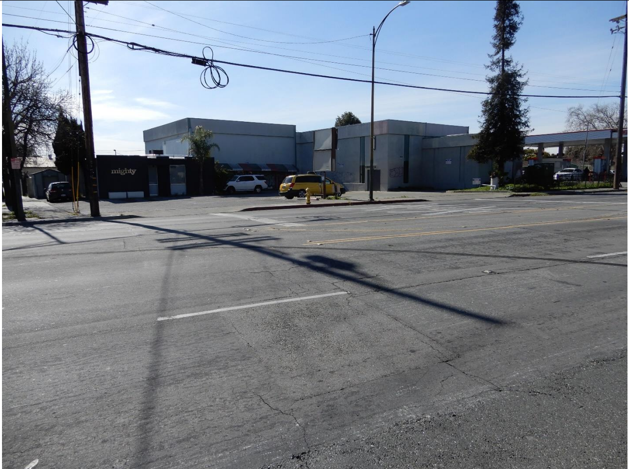
1266 E. Julian Street (1987), on the south side of E. Julian Street across from the subject properties, view southwest (ARG, March 2021)
