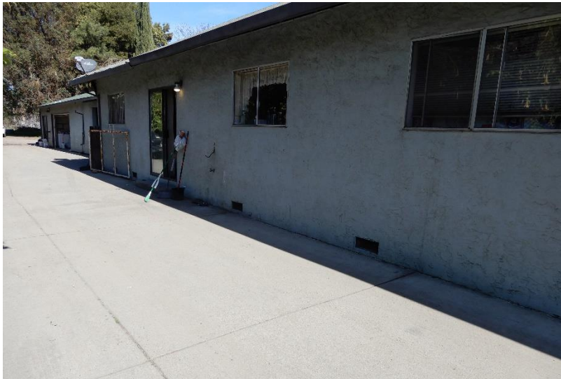
Figure 3. 1271 E. Julian Street, west façade, view northeast (ARG, March 2021)
