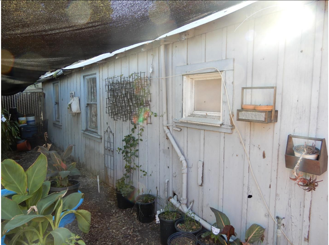
1279 E. Julian Street, one-story residential building, partial view of north façade, view southeast (ARG, March 2021)
