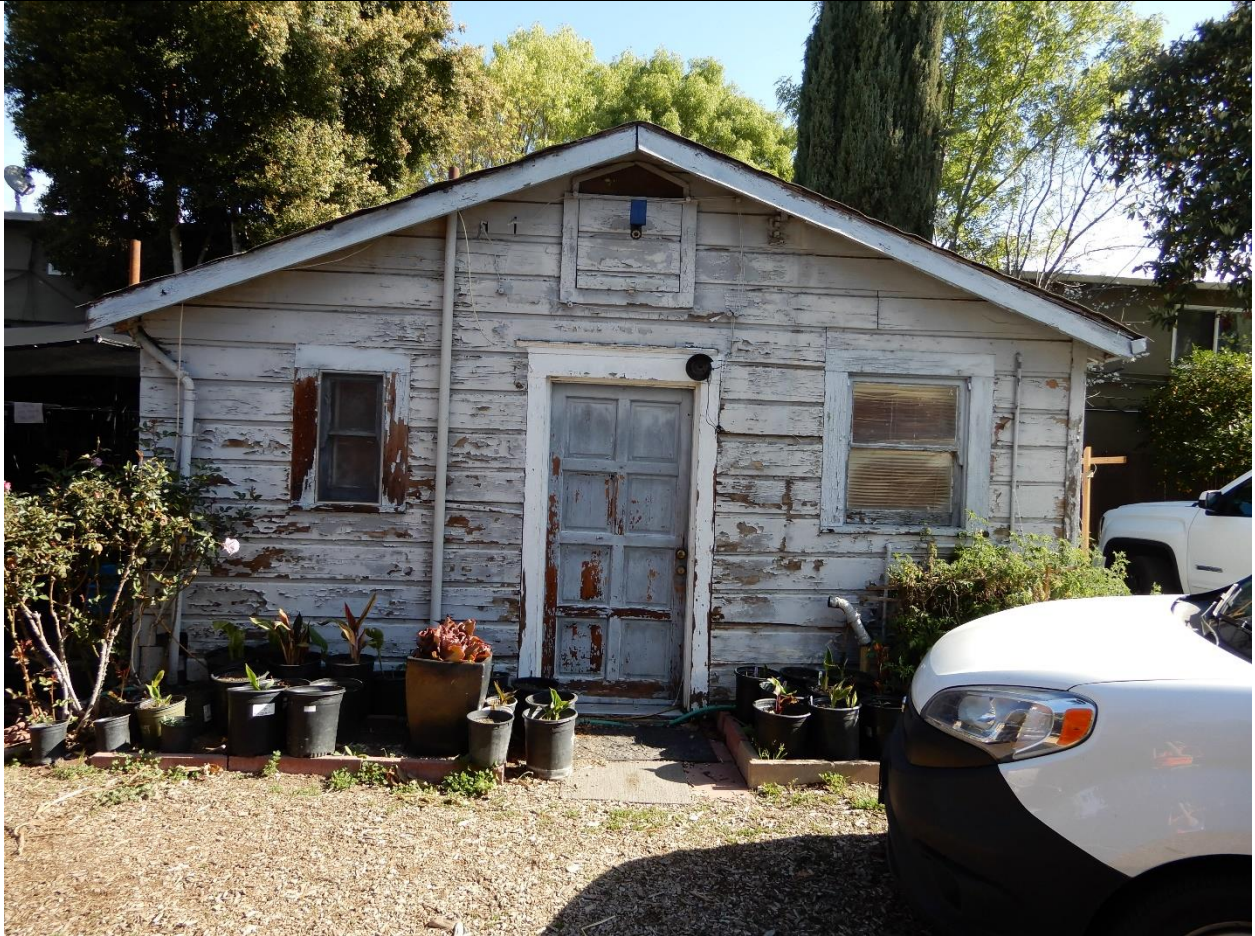
1279 E. Julian Street, one-story residential building, west façade, view east (ARG, March 2021)
