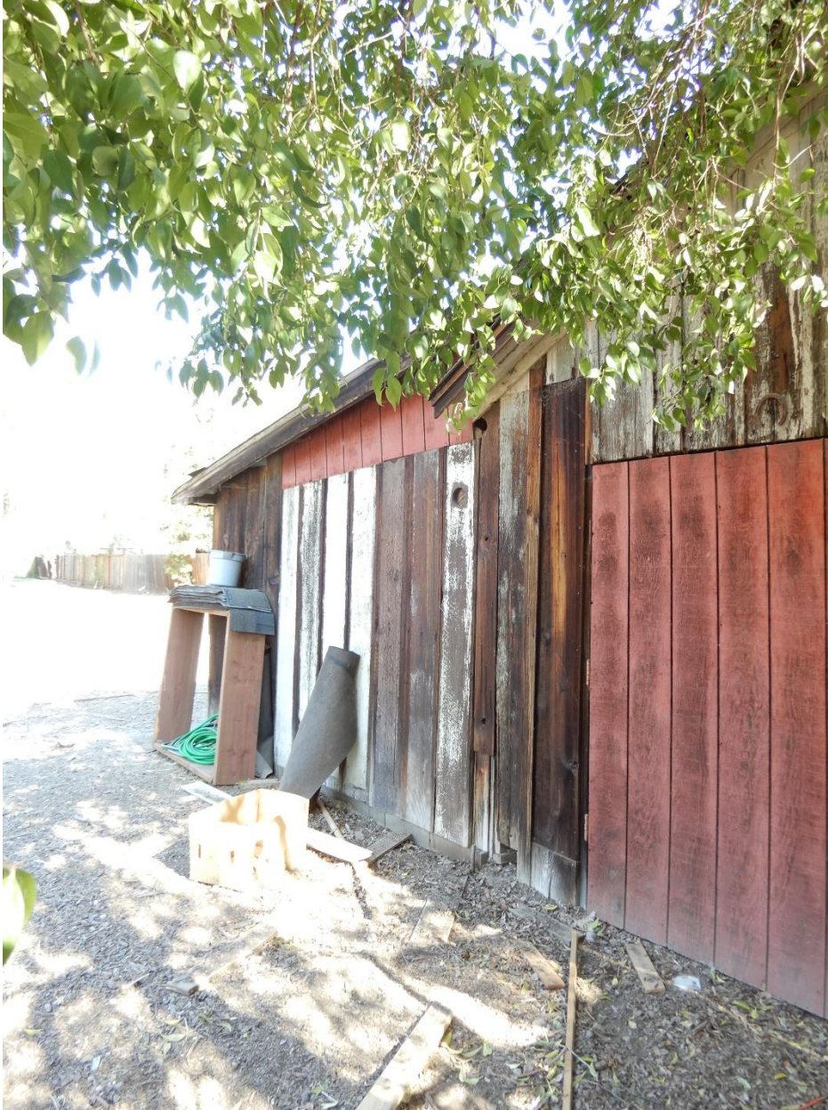
1279 E. Julian Street, one-story structure, west façade, view northeast (ARG, March 2021)
