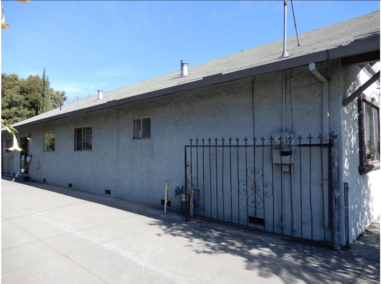
1271 E. Julian Street, west façade, view northeast (ARG, March 2021)
