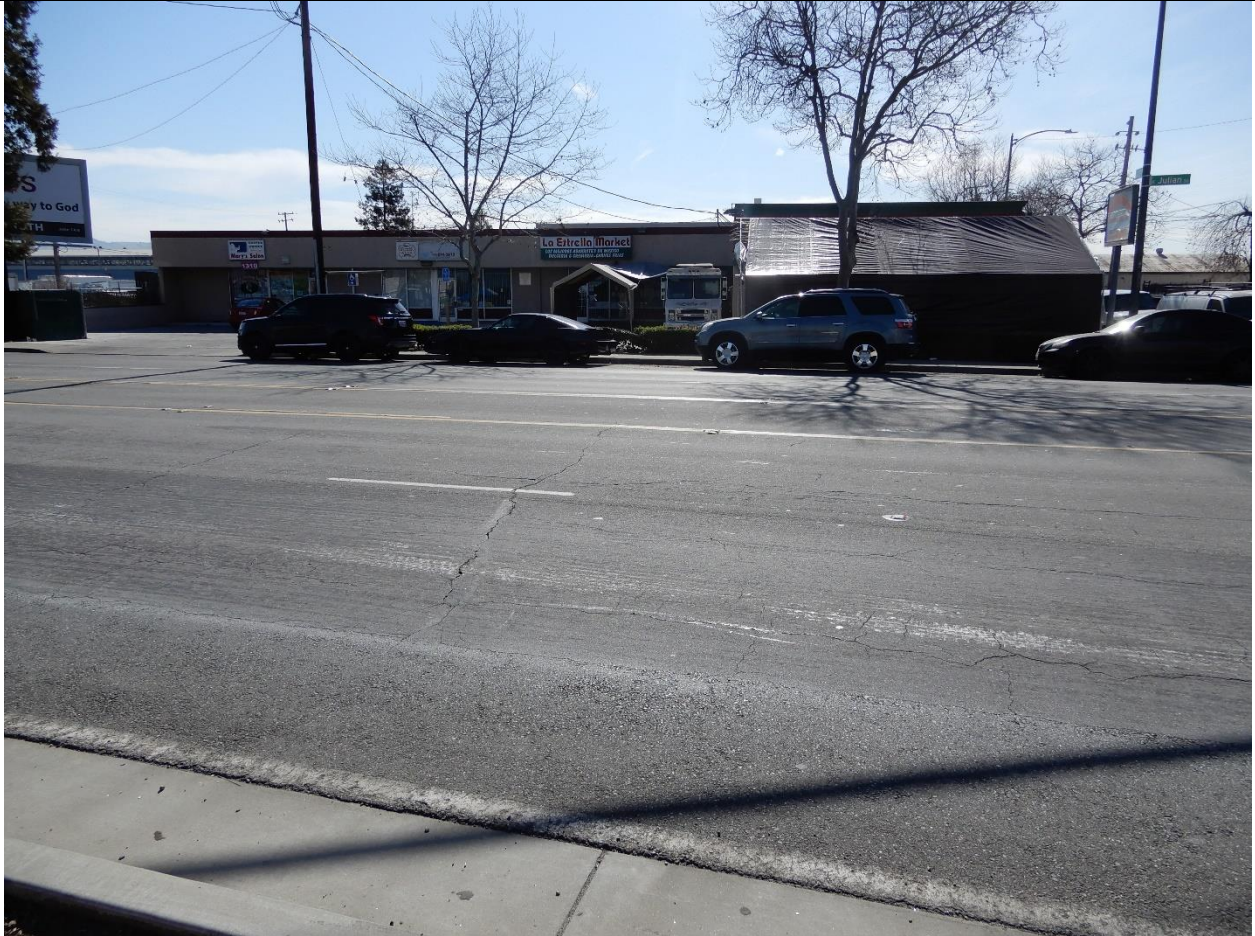
1272 E. Julian Street (1965), on the south side of E. Julian Street across from the subject properties, view south (ARG, March 2021)
