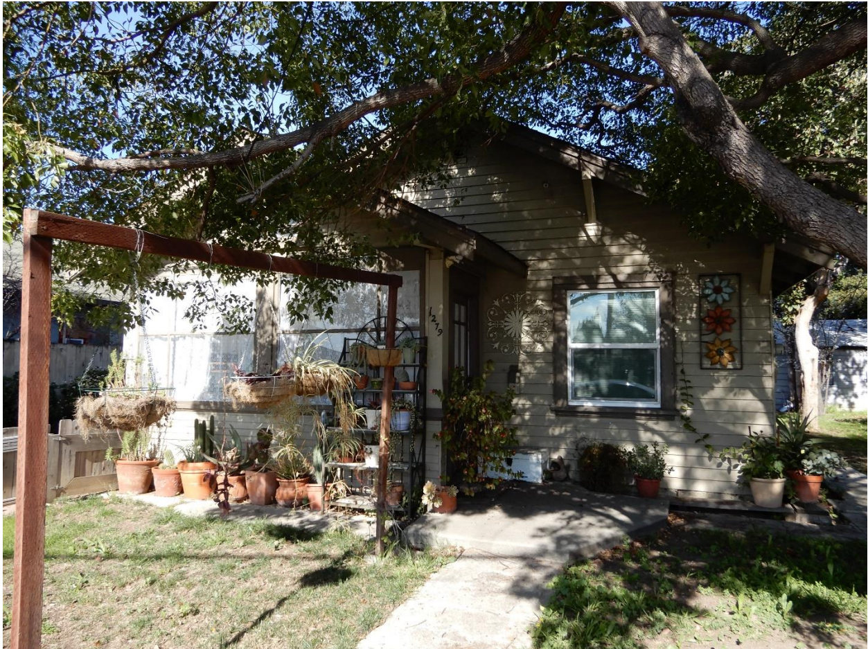
1279 E. Julian Street, primary (south) façade, view northwest (ARG, March 2021)
