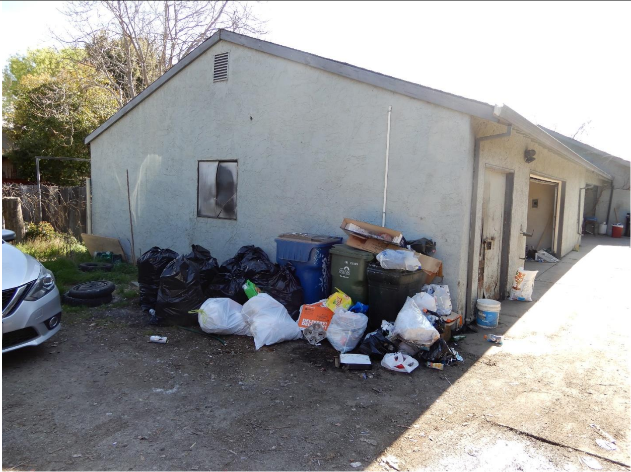
1271 E. Julian Street, rear (north) façade, view southeast (ARG, March 2021)
