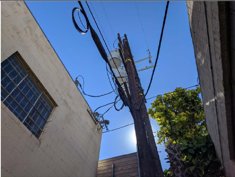
**PHOTO 6:** View of pole-mounted transformers along the east boundary of the Site.
