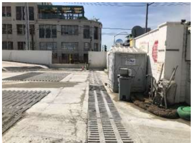
18. View south at the western portion of the Site.
