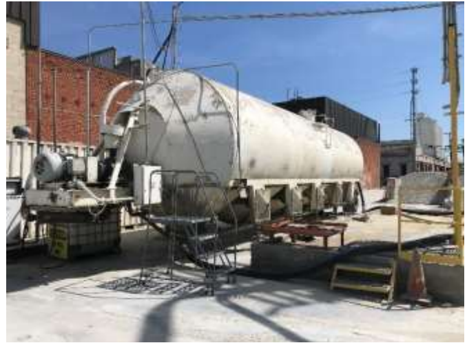
20. Eastern adjoining cement chemical storage tank.
