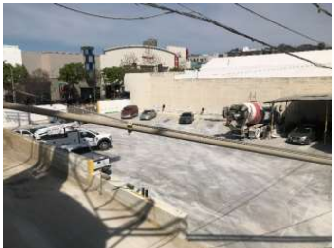
6. View northwest of the northern portion of the Site.
