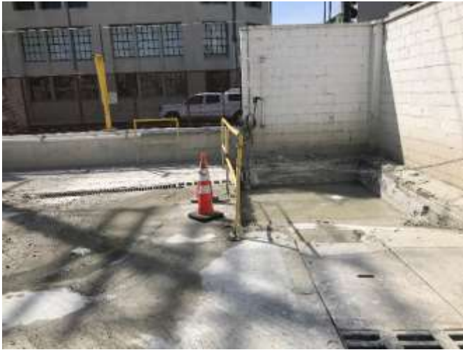
7. View of surface drain and collection basin at the southwest corner of the Site.
