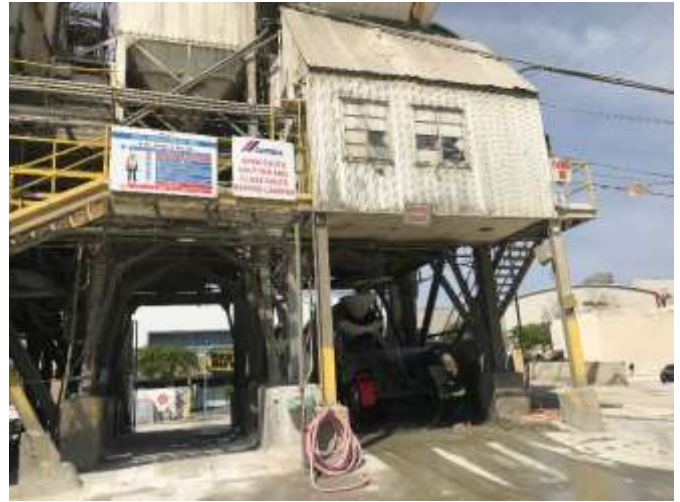
8. View west of the cement mixing tower.
