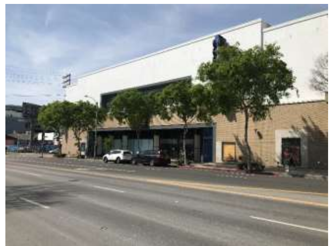
24. Western adjacent retail center.
