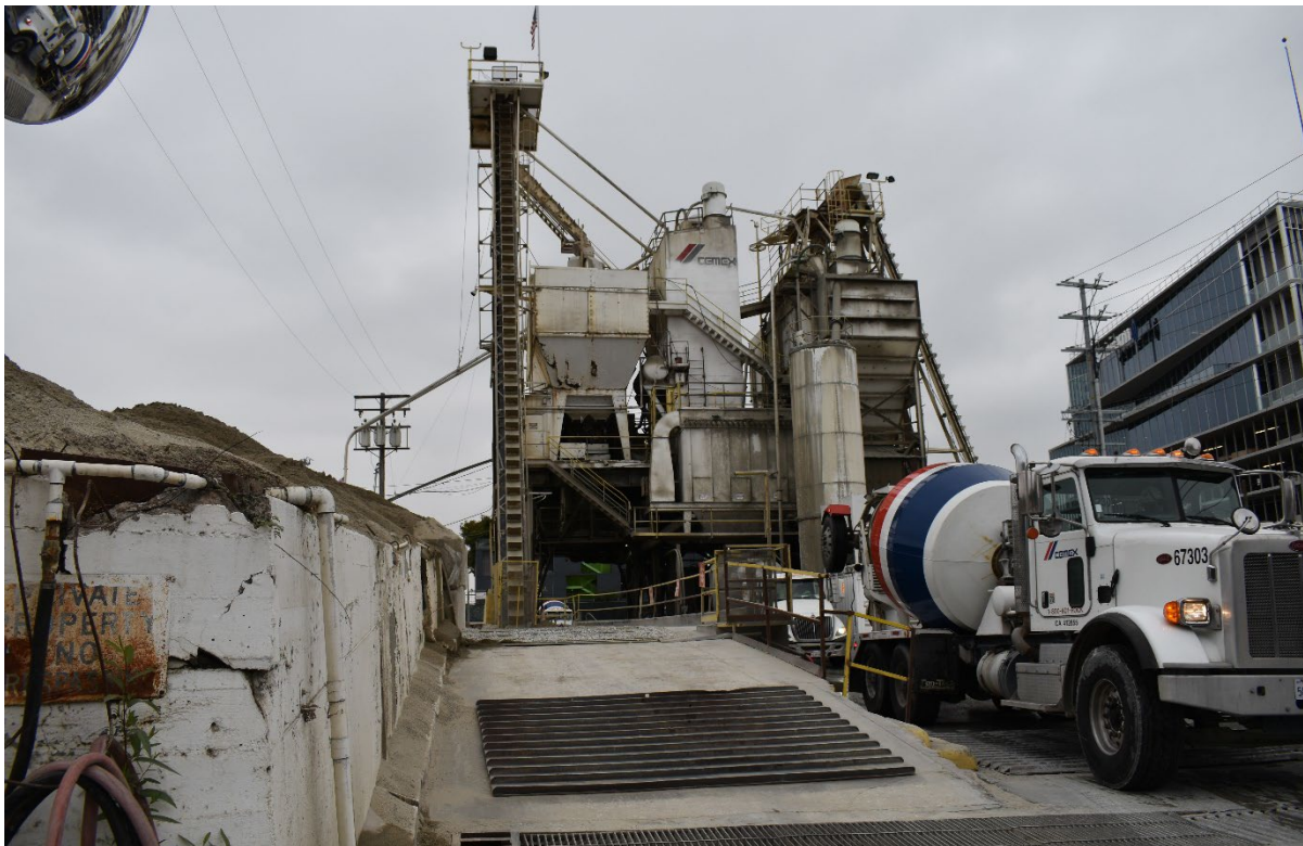
Figure 4 View of the On-Site CEMEX Concrete Plant from North La Brea Avenue
