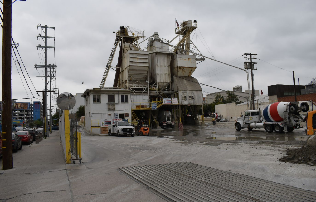
Figure 5 View of the On-Site CEMEX Concrete Plant from Romaine Street
