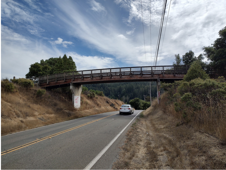
Figure IV.1-3: Bridge over Nicasio Valley Road
