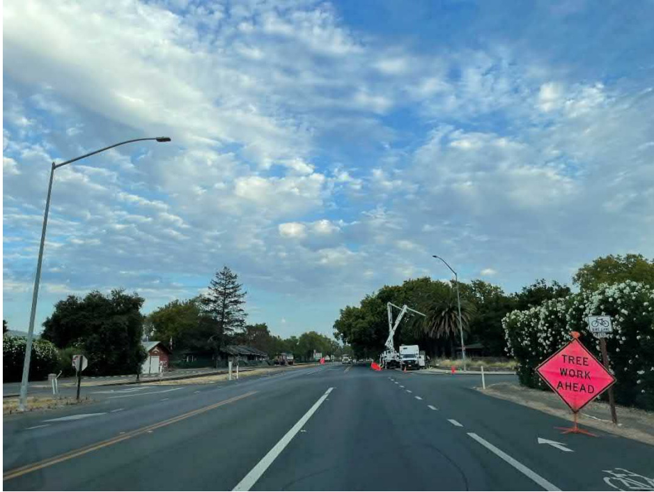
Photo 1: Project site, facing northwest at intersection of SR-29 and Rutherford Rd.
