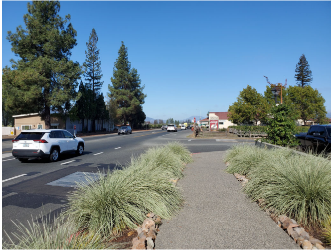
Photo 1 – Oakville Cross Road/SR-29 Intersection, looking north
