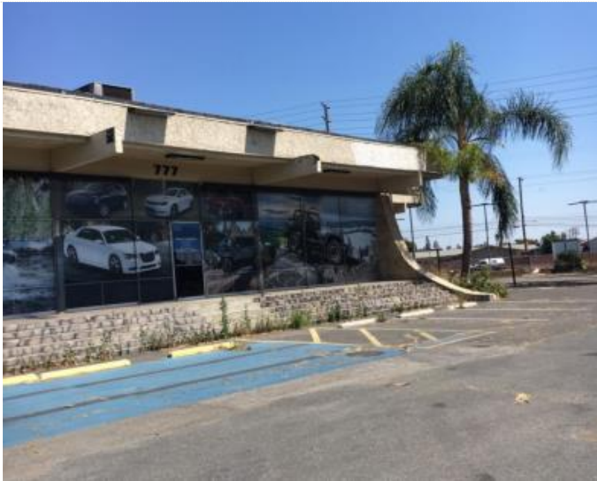
Photo #1: Exterior of Showroom
