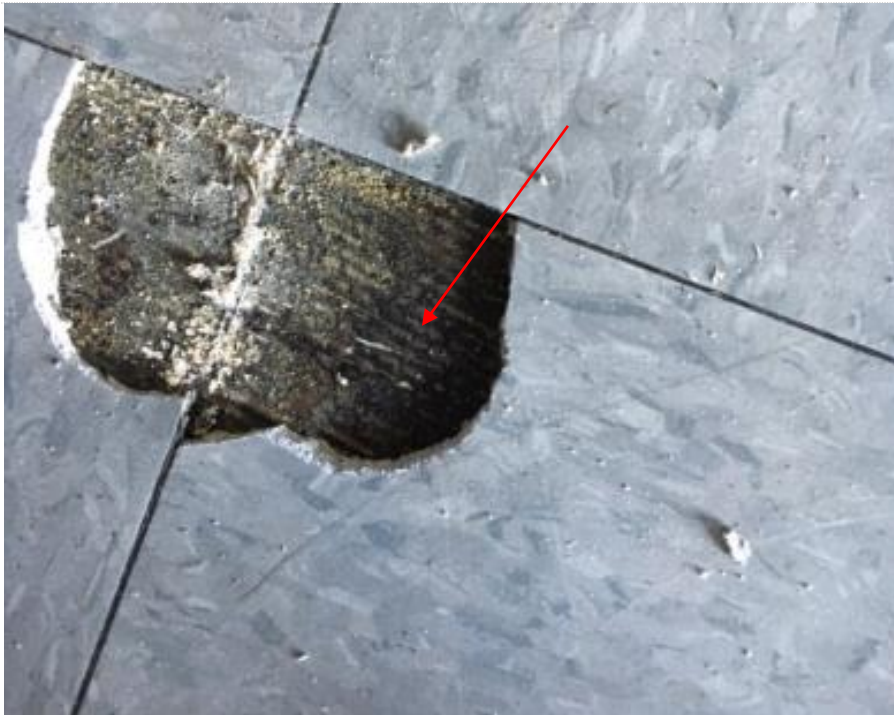
Photo #5: Photo of sample group 0603-08 (12x12 gray floor tile) and positive sample group 0603-09 (black mastic),
