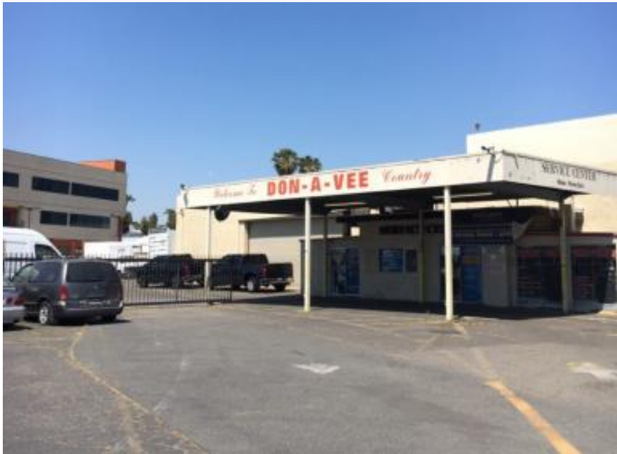
Photo #2: Exterior of Service Center
