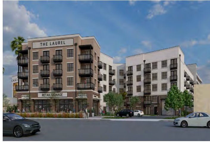
VIEW ON ORANGETHORPE AVE LOOKING NORTH 2
