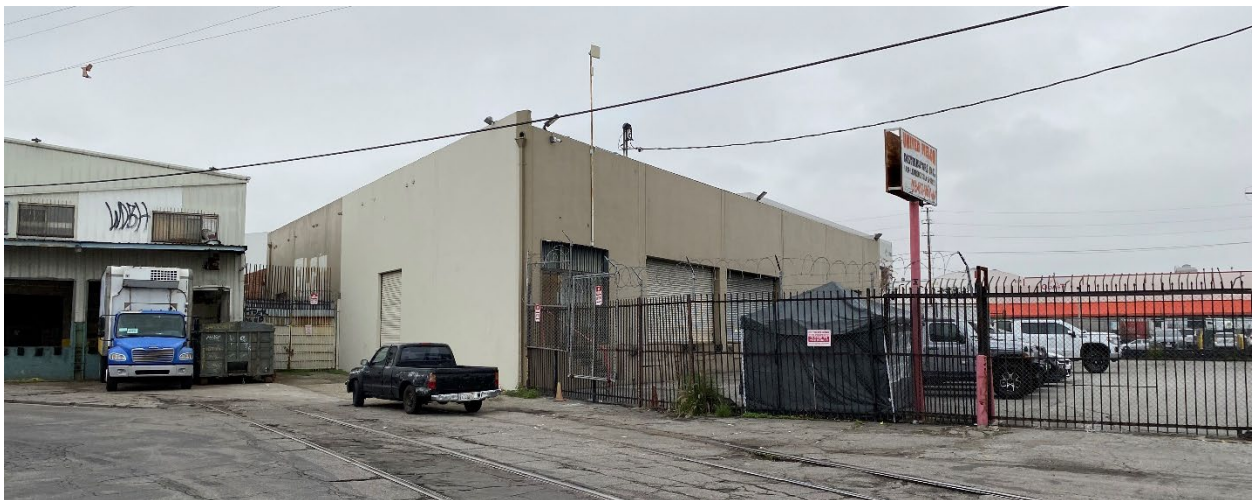
Photograph 4. View of 1811 Sacramento Street, looking northwest (Stantec December 2022).
