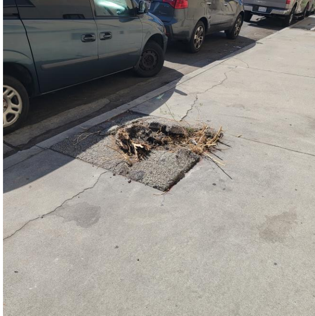
Shown is the remaining stump from a previously removed street tree
