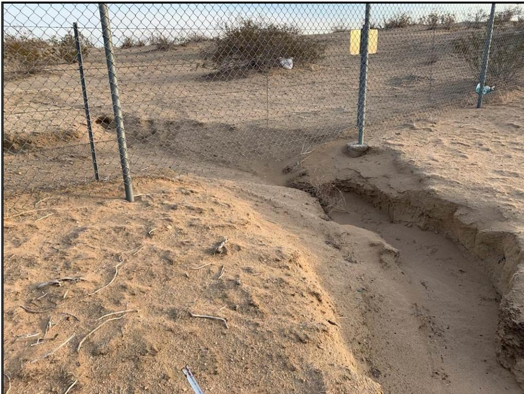
Photo 6: Deteriorated Desert Tortoise Fencing Along Northern VVWRA Facility; Facing North.
