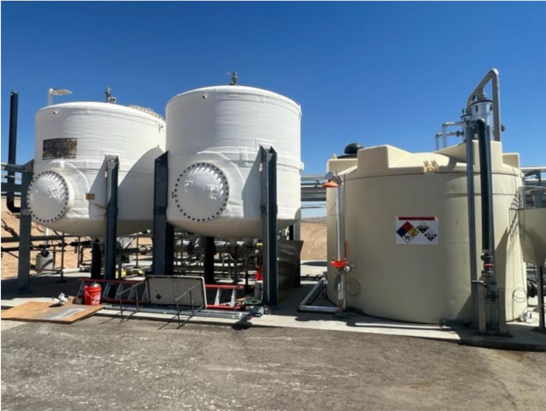
Biogas Upgrading System - 93% Sulfuric Acid Tank (5,400 gallons)
