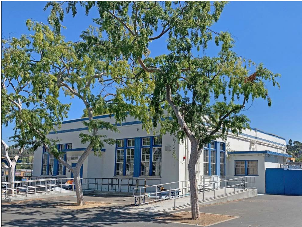
Figure 64. Windows on Cafeteria building. Shows two-light section above two-by-four-light section, with fluted plaster piers separating window pairs.
