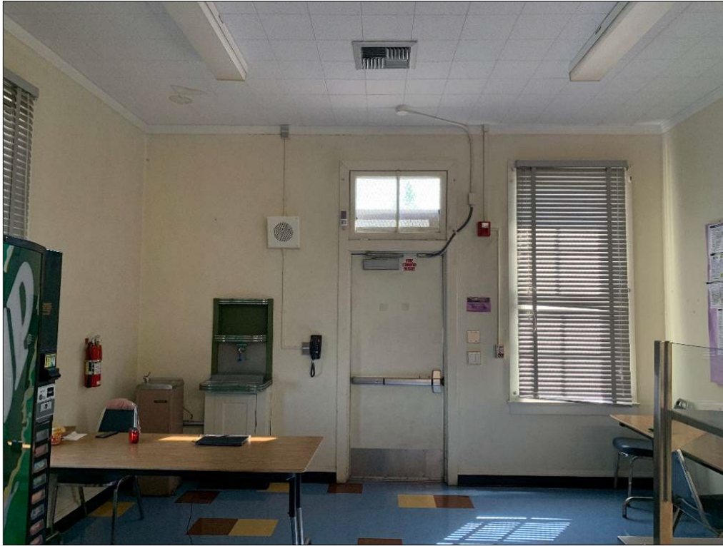
Figure 66. Two-light transom and Moderne-style water station in Faculty Dining Room in Cafeteria.
