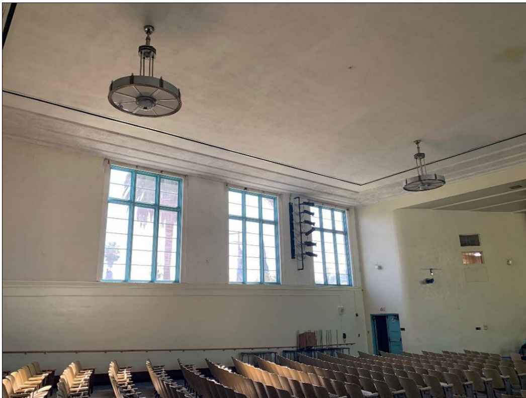
Figure 45. Interior view of windows at northeast façade of Auditorium.
