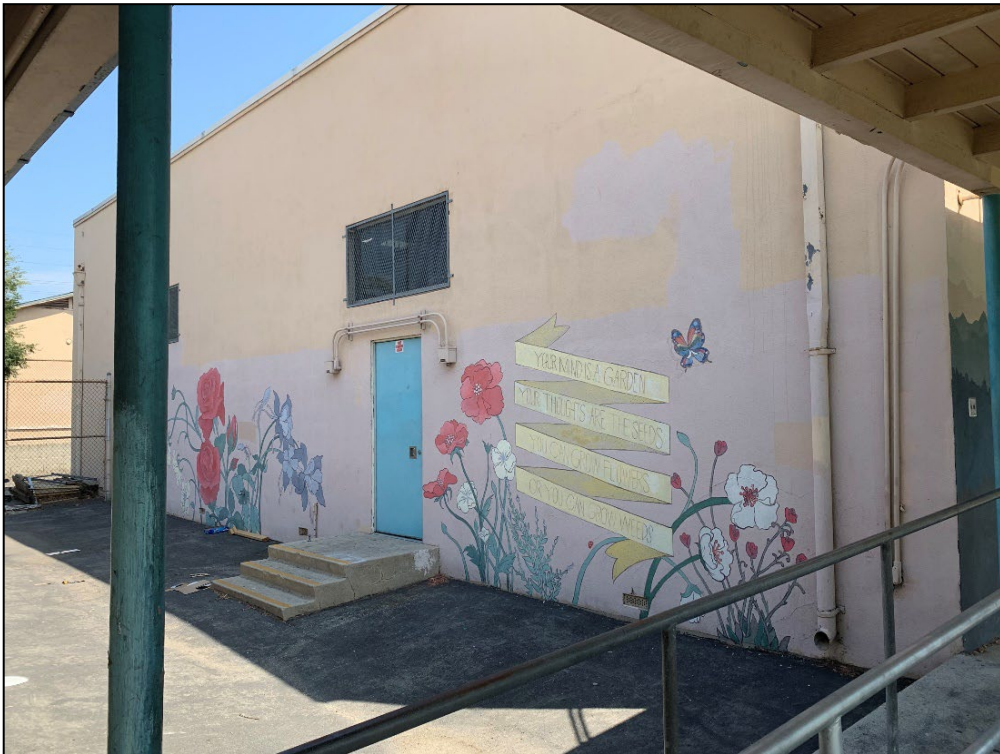
Figure 70. Southwest façade of Shop No. 1, view toward the east.
