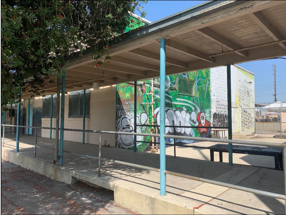
Figure 69. Corridor connecting the two Shops, view toward the west.
