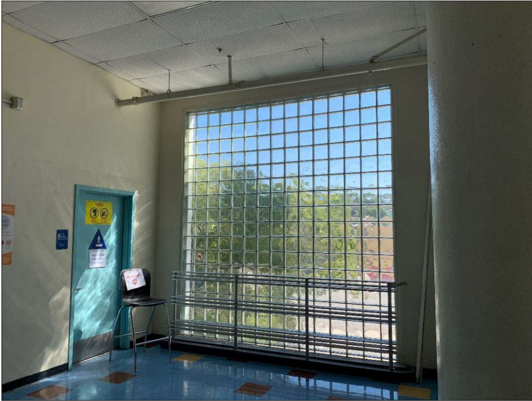
Figure 20. Interior view of glass-block wall at northeast end of Administration Building.
