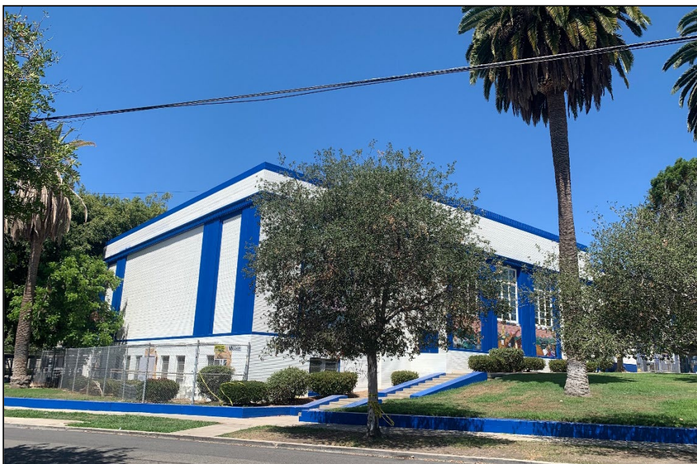
Figure 38. Southeast and northeast façades of the Auditorium, view toward the west.
