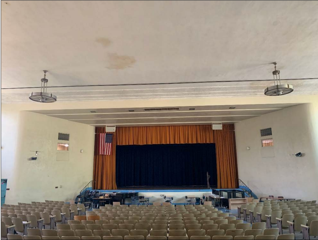
Figure 42. Stage, curved walls with stepped ceiling, raked seating, and chandeliers in Auditorium, view toward the southeast.
