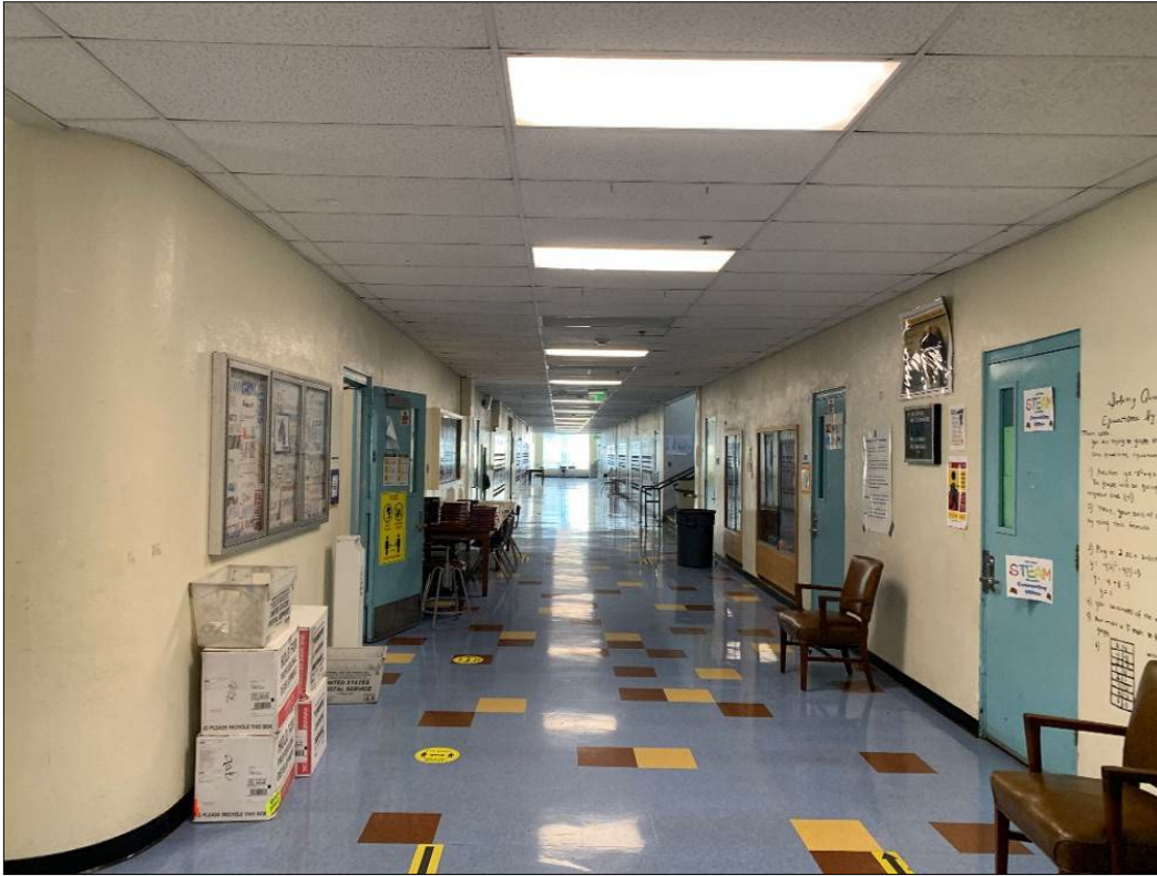
Figure 25. Rounded corner wall in the corridor of the Administration building.
