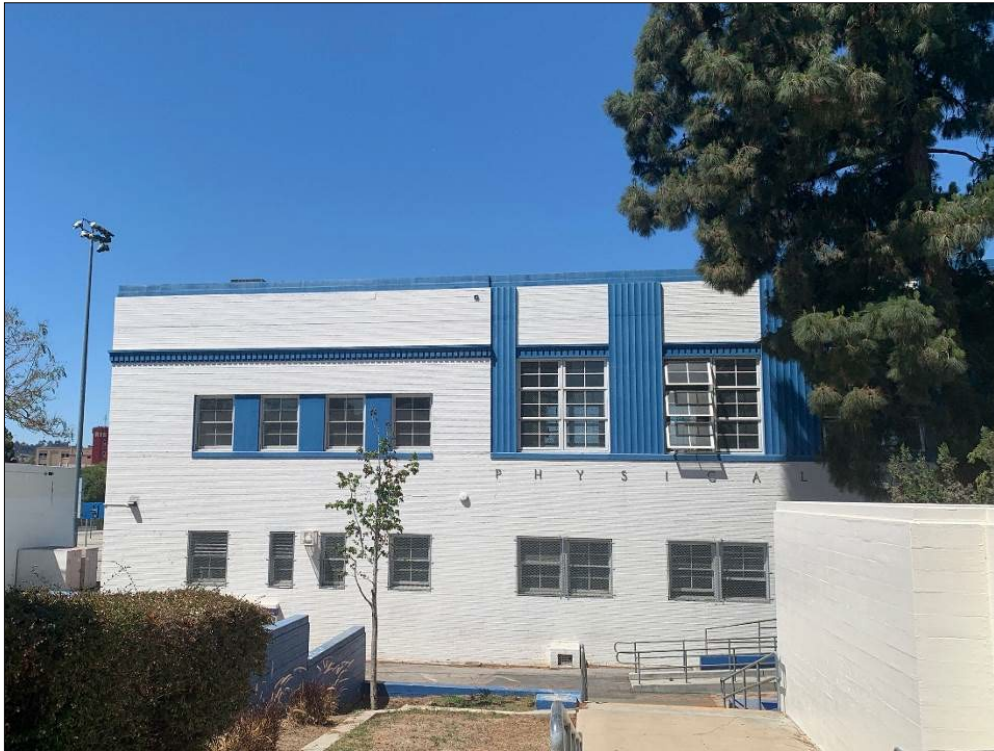
Figure 55. Window configurations at northeast (primary) façade of Physical Education Building.
