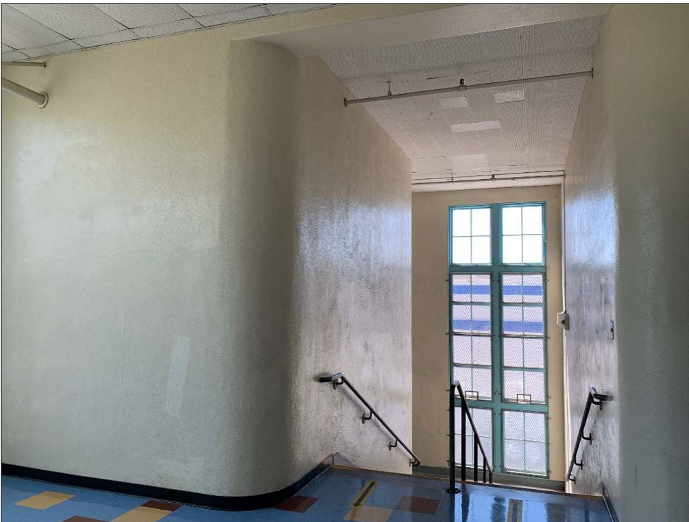
Figure 26. Rounded corner wall and vertically oriented multi-light window in stairwell.
