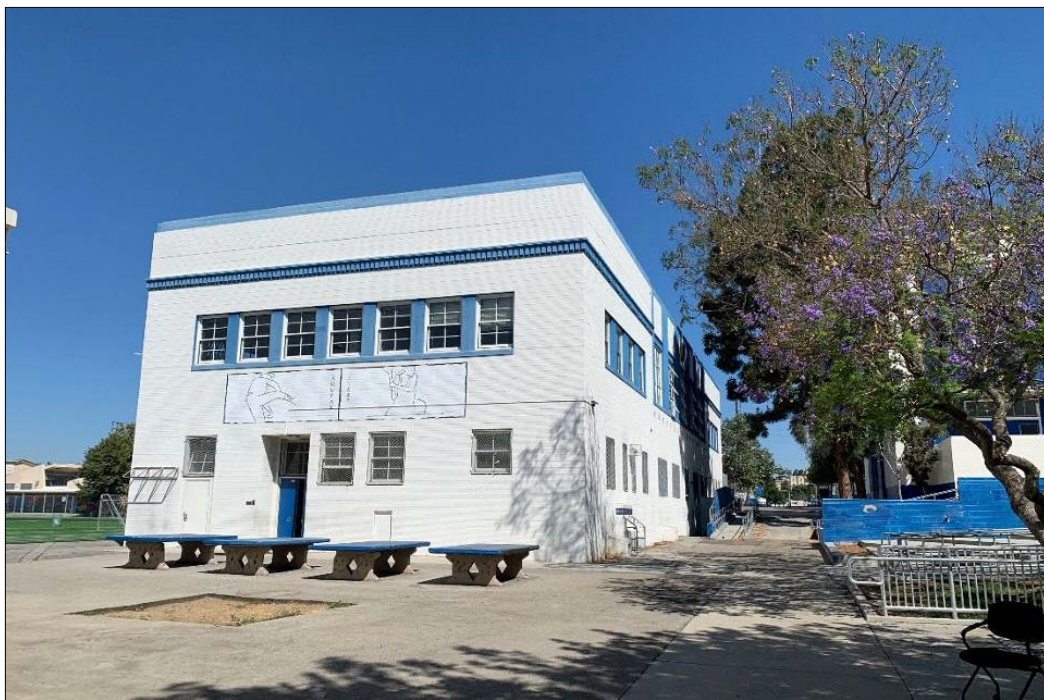
Figure 54. Physical Education Building, southeast façade. Shows dentil molding below parapet and arrangement of windows.
