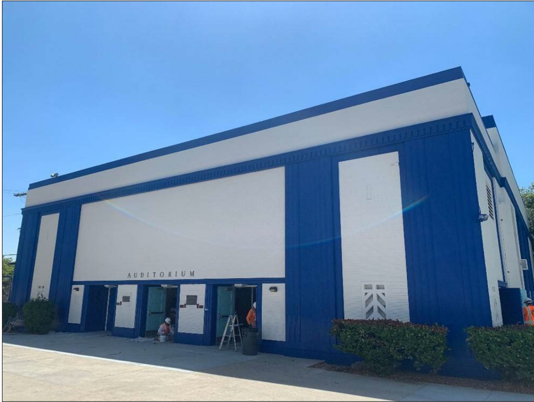
Figure 29. Northwest (primary) façade of Auditorium. Shows fluted pilasters, stringcourses, and primary entrance.
