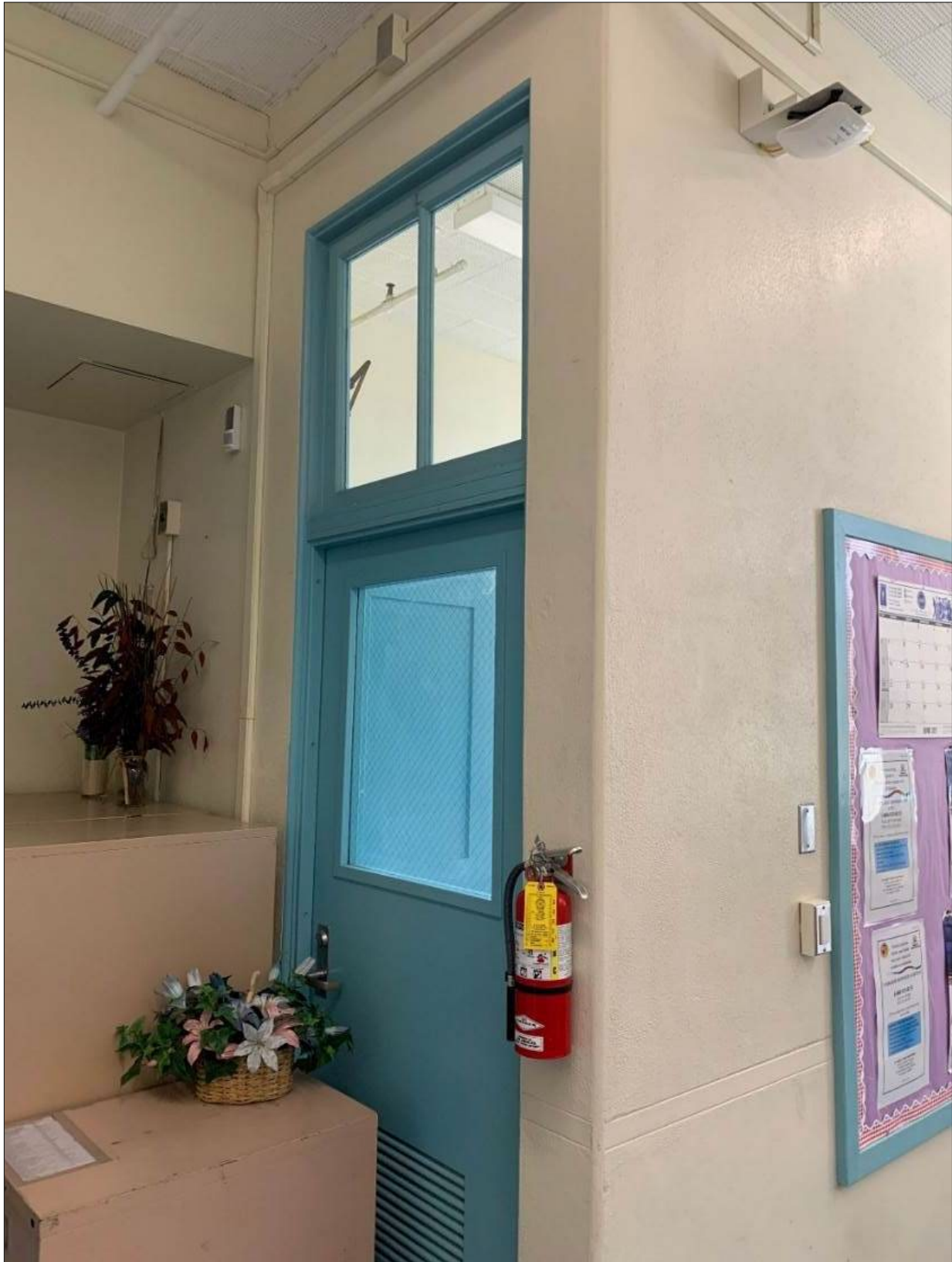
Figure 23. Two-light transom in Administration Building.
