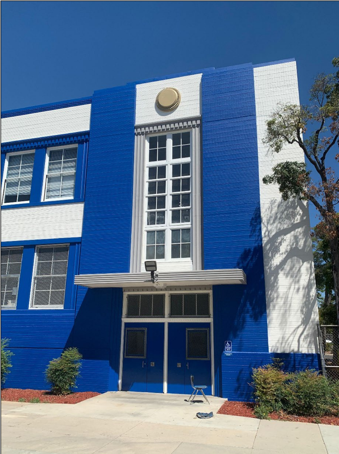
Figure 12. Secondary entrance at southeast façade, showing horizontal board-formed concrete texture on exterior walls.
