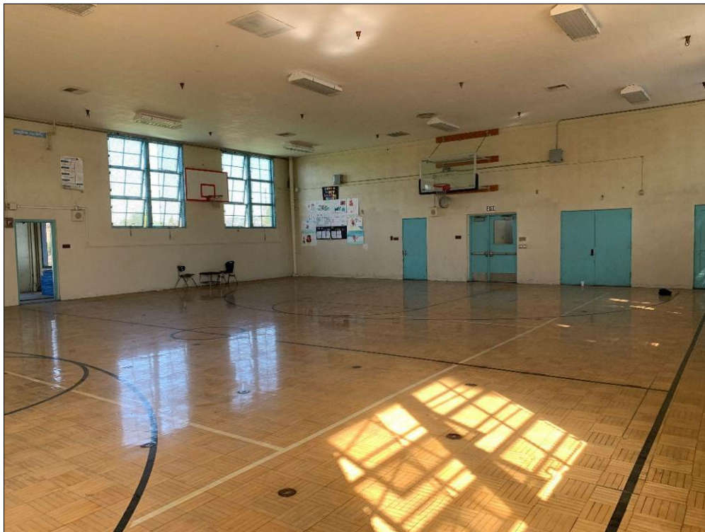
Figure 61. Parquet wood floor and awning-type windows in gymnasium of Physical Education building.
