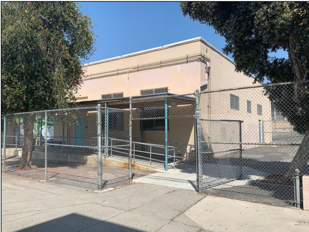
Figure 72. Southeast and northeast façades of Shop No. 2, view toward the west.
