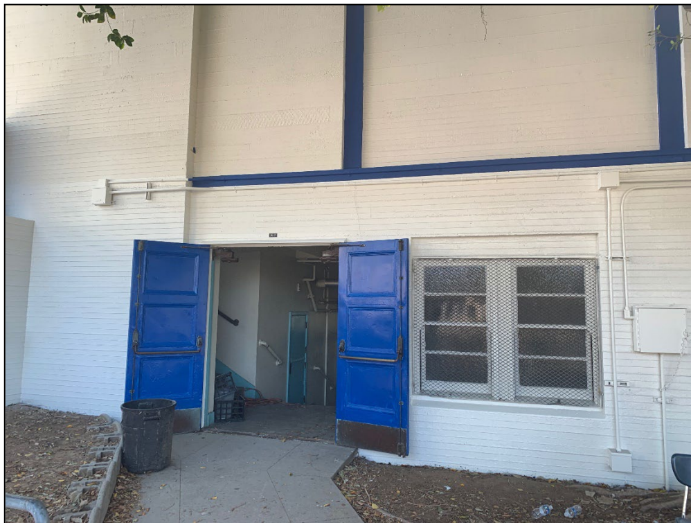
Figure 36. Entrance on the southwest façade at lower level, view toward the northeast.
