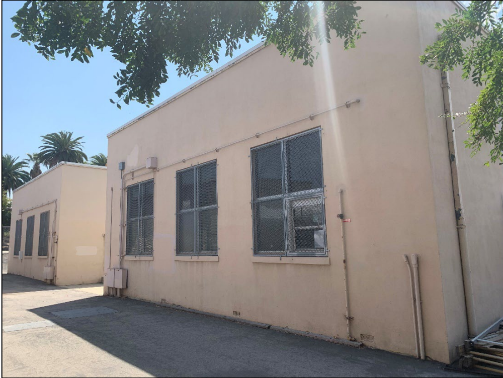
Figure 71. Northwest façades of shops, view toward the east.
