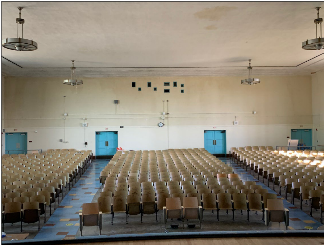
Figure 43. View of assembly hall from stage, looking southeast.
