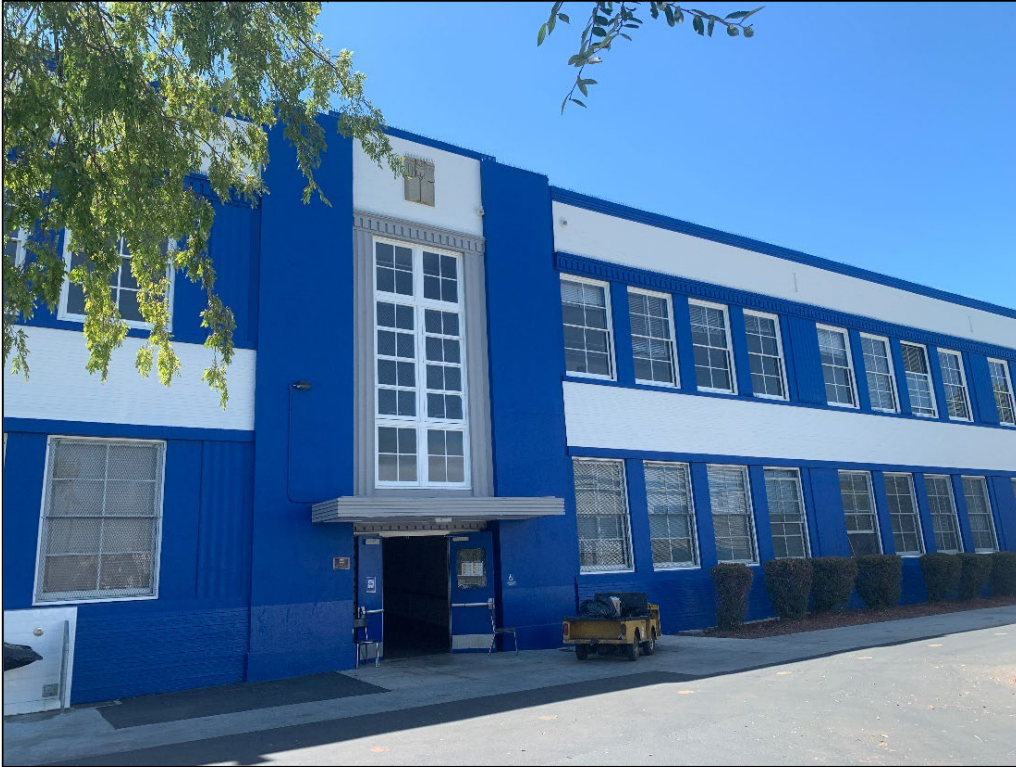
Figure 16. Center of the northwest façade, view toward the south.
