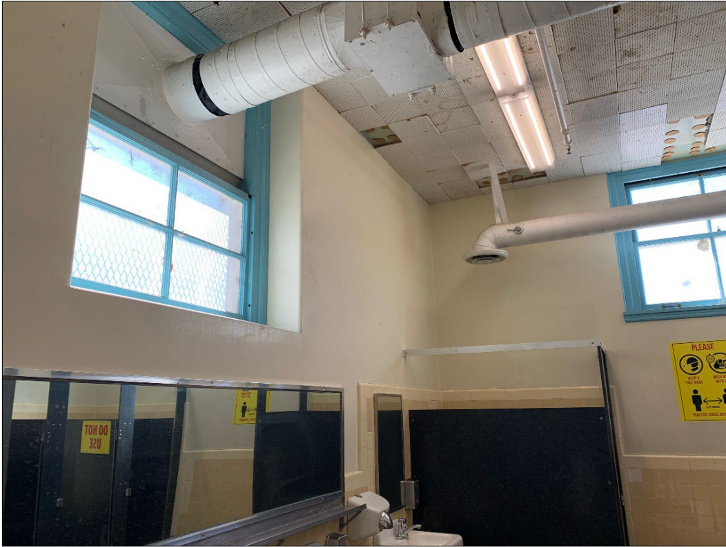
Figure 56. Interior of locker room on first floor, view toward the southeast.
