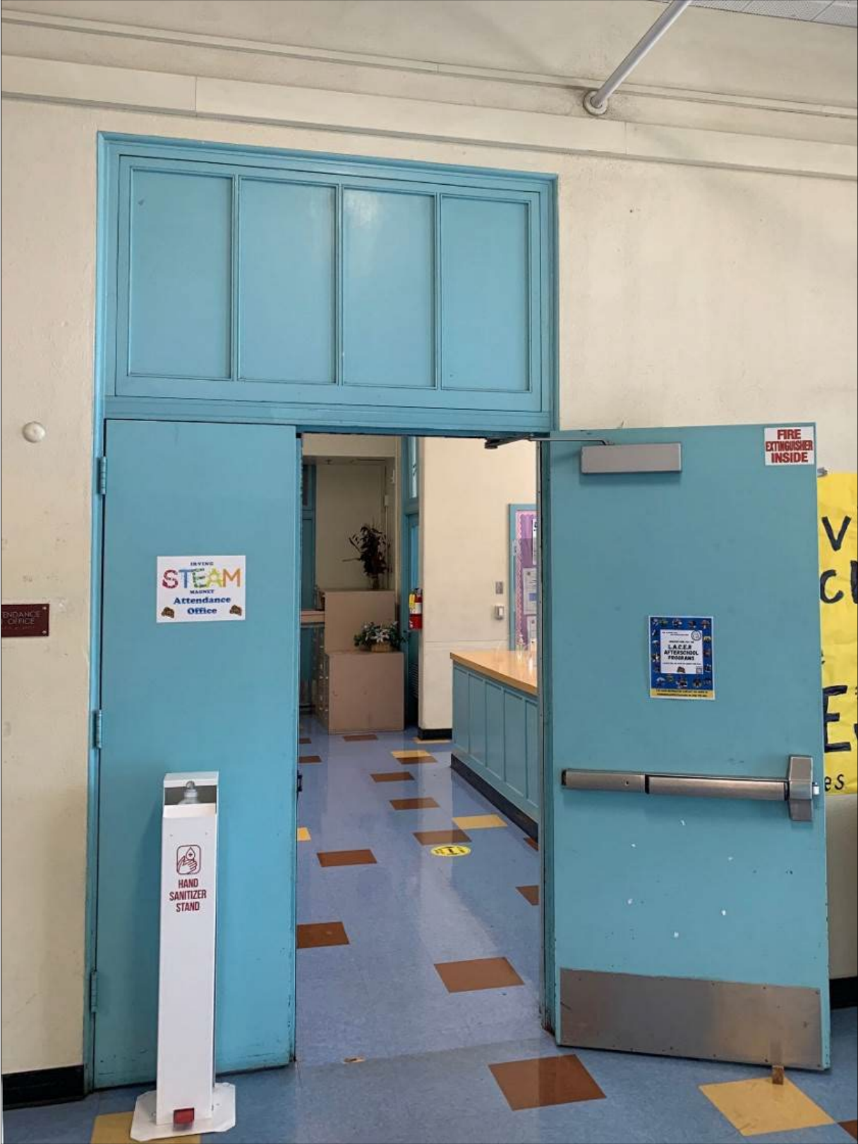
Figure 24. Four-light transom in Administration building.
