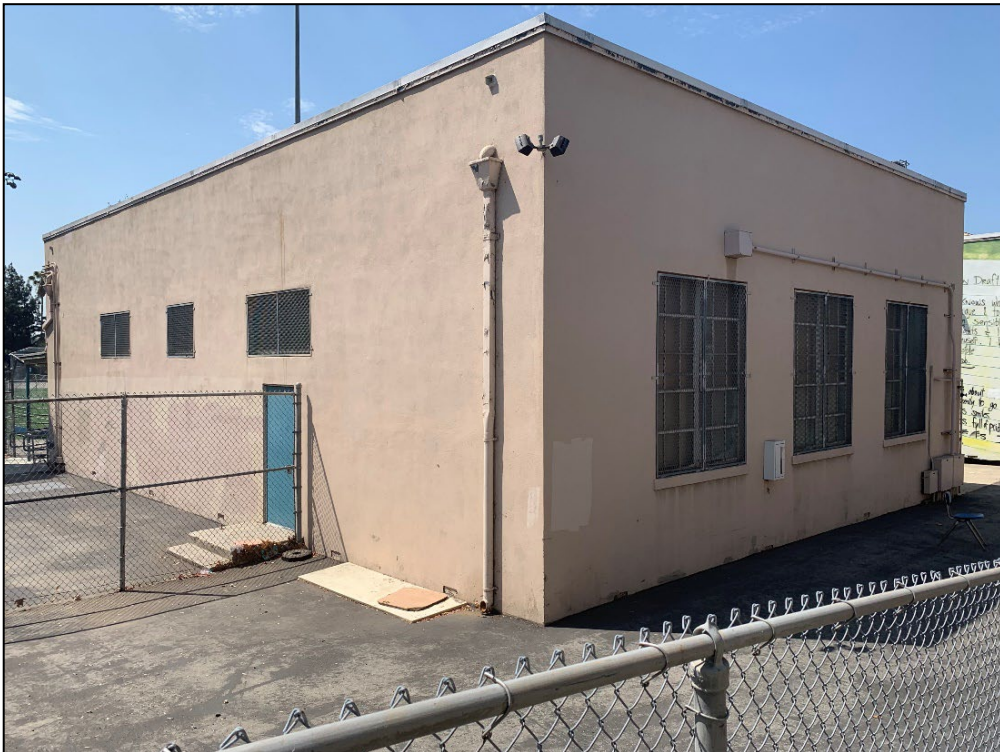
Figure 74. Northeast and northwest façades of Shop No. 2, view toward the south.
