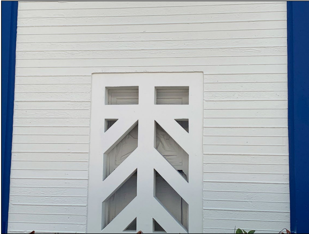
Figure 31. Detail of concrete grille on secondary windows and detail of board-form concrete texture.
