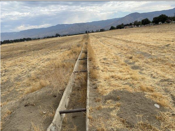
View of concrete lined former irrigation channel
