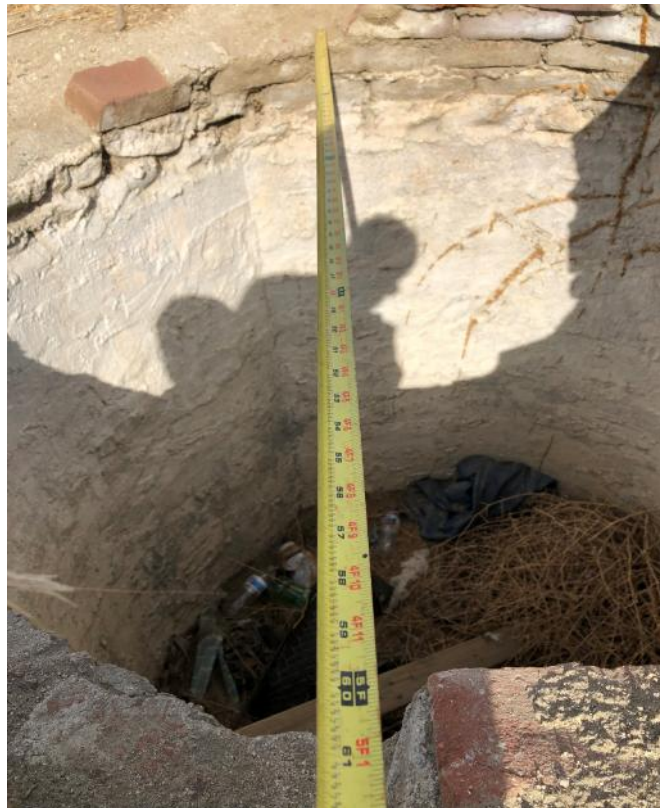
Photograph No. 14: Open cylindrical excavation (shaft) in southwest portion of site is about 5 feet in diameter
