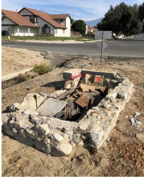
Photograph No. 5: Rectangular-shaped concrete structure filled with debris in northeast corner of site near the intersection of Karon Street and Pennsylvania Avenue
