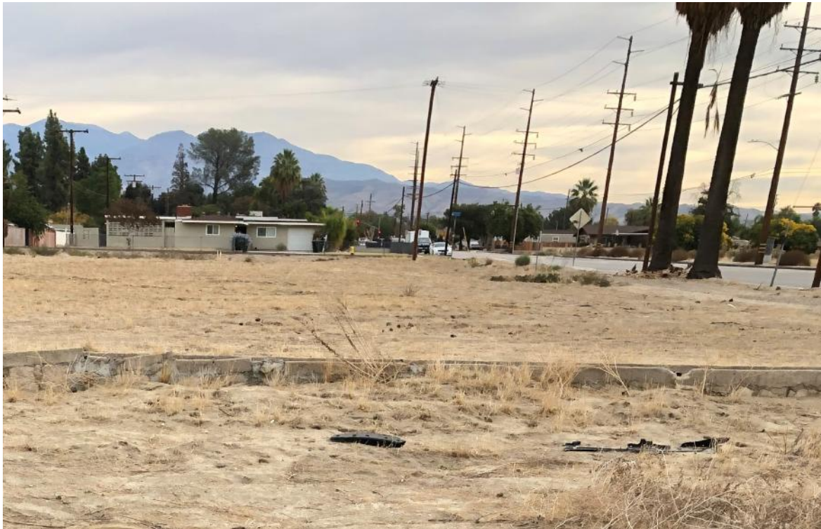
Photograph No. 2: Viewing east at U-shaped concrete structure (electrical easement) that trends in a north-south orientation across the south-central portion of the site
