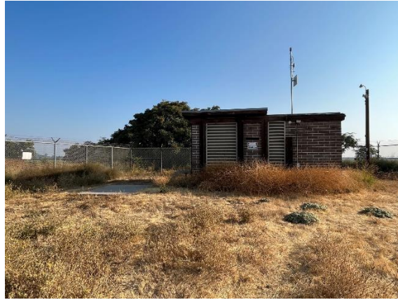
Photo 2 - Pump house building.
