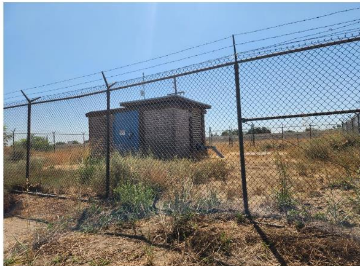
Photograph 2. Well house facing south.
