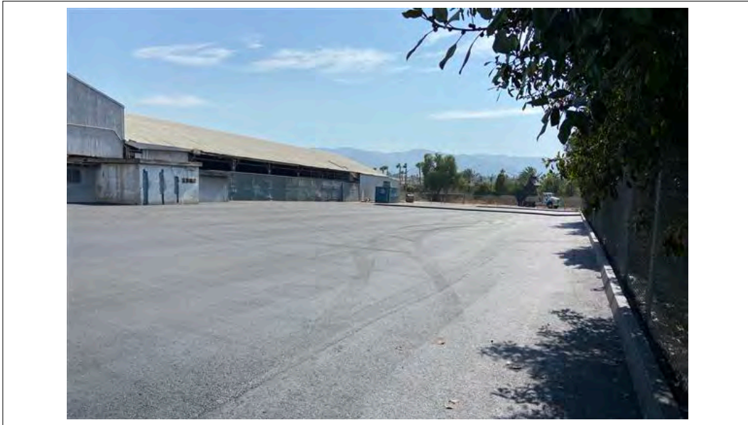
View from northeast corner of AOC1 with pavement and associated curbing (9/9/21).
