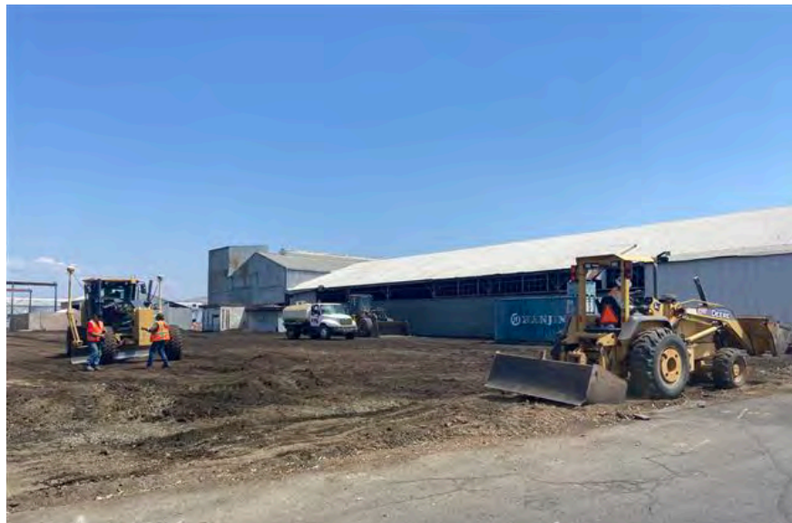
View from northwest side of AOC1. View of ripping and moisture conditioning activities up to the edge of the current asphalt pavement after fencing was removed. (8/31/21)
