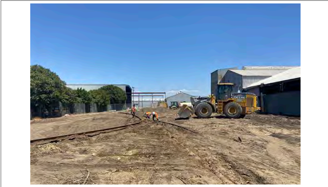
View of AOC1 from west boundary. View of railroad removal activities (8/4/21)
