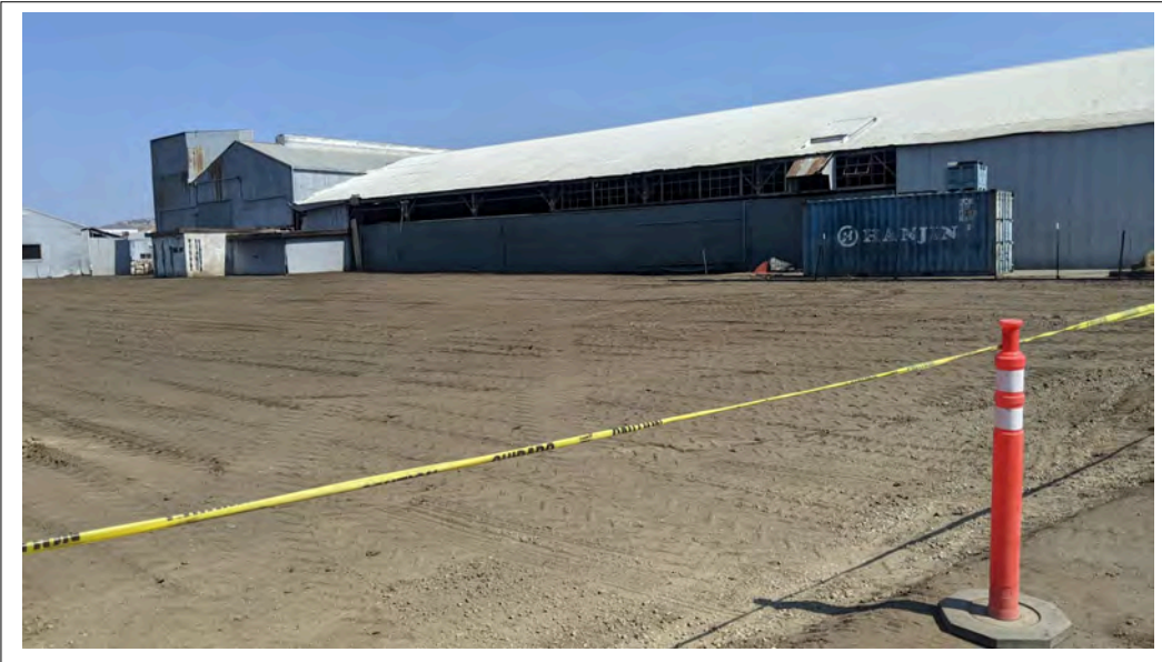
View of AOC1 from west side prepped for paving (9/7/21)
