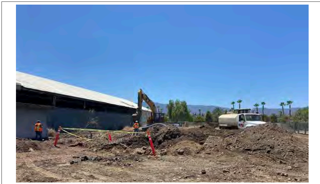
View from AOC5 east side facing west. View of excavation activities associated with former septic tank debris/piping (8/3/21).
