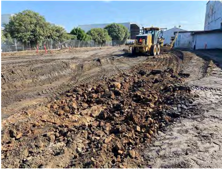
View from southwest corner of AOC1 facing east. View of ripping activities (8/30/21)
