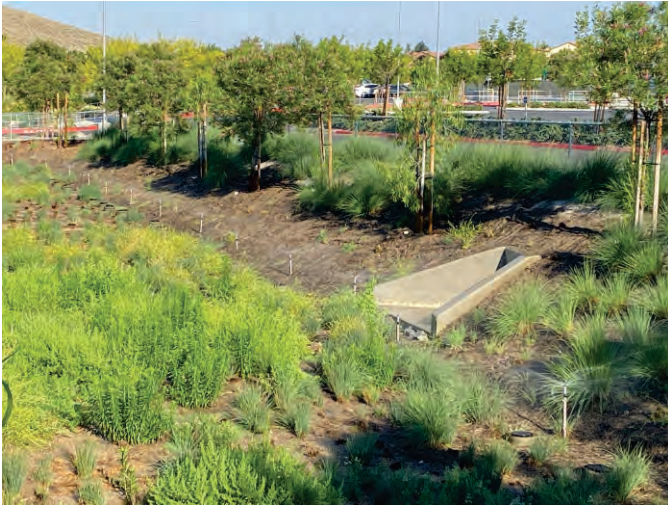
Photo 9: View looking west at Detention Basin 6 located on the northwestern corner of Skyview Road and Washington Street.
