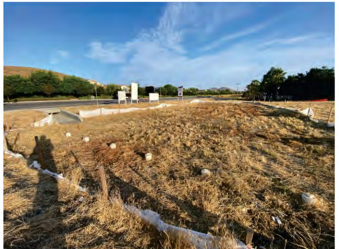
Photo 8: View looking west at Drainage D located on the northeastern corner of Autumn Glen Circle and Washington Street.
