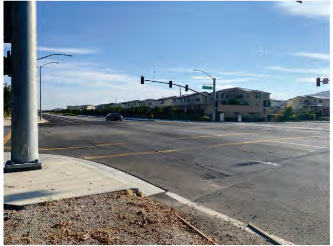
Photo 10: View of the southern project boundary looking north at the Skyview Road and Washington Street intersection.
